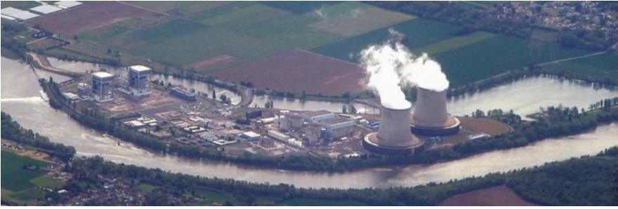
Photo 2.78 Saint-Laurent-des-eaux site. The two Natural Uranium-Graphite-Gas (UNGG) reactors are located at the far left, recognizable by their cubic shape. Two air-cooling towers in operation are located at the end of the site on the right. The two PWRs that they cool in addition to the Loire River are located just to the left of the towers, recognizable by the hemispherical shape of the reactor buildings and the next large parallelepipedal turbine buildings
