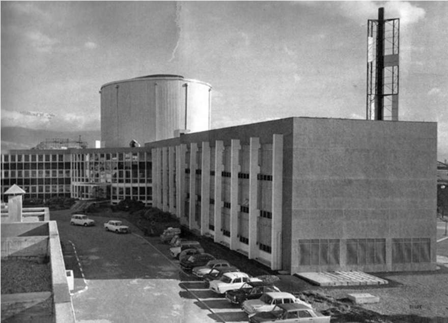
Photo 2.52 Siloé building inside the CEA site. The reactor is located in the white cylindrical building
