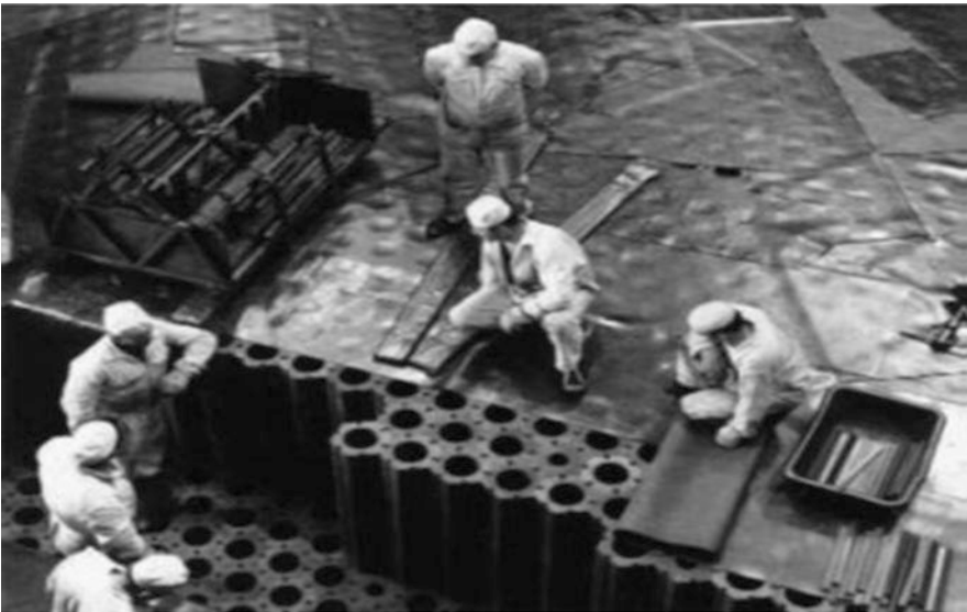
Photo 2.80 Building the graphite pile: channels through the graphite sleeves are clearly visible
