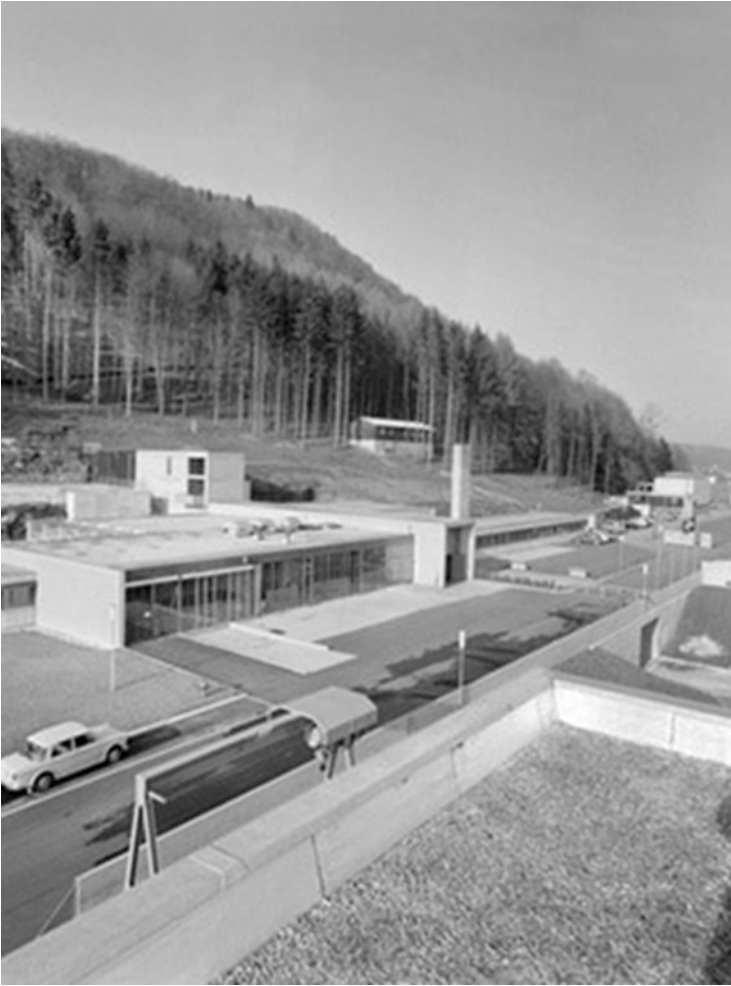
Photo 2.60 The surface buildings of Lucens in 1969
