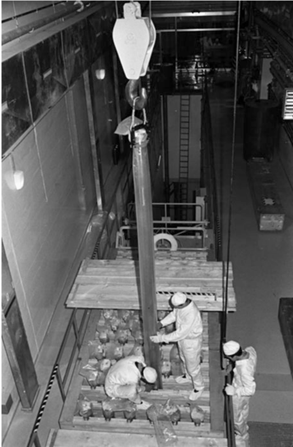
Photo 2.64 Placing a fresh fuel assembly in a storage rack. The core contains 73 such assemblies. The spent fuel assemblies are evacuated without contact by the unloading machine to the deactivation pool
