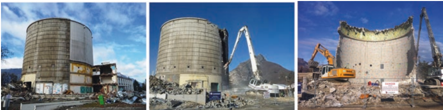
Photo 2.56 Dismantling of the Siloé reactor building (CEA-Grenoble) (photo Cardem and Eurovia-Vinci)
