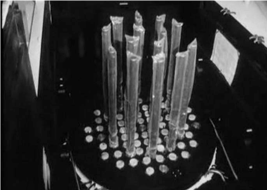
Photo 2.67 View of the upper side of the Lucens reactor vessel (photo IFSN). The control rods and shutdown control rods, wrapped in transparent plastic, can be seen emerging from the vessel cover
