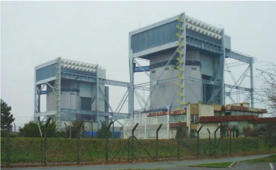
Photo 2.79 The two reactor blocks of Saint-Laurent-A1 and A2. The welded structures that surround them are characteristic of the French Natural Uranium-Graphite-Gas (UNGG) of the late 1960s
