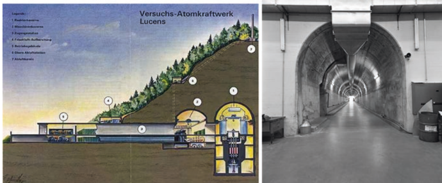
Photo 2.61 The access tunnel to the cavern reactor
