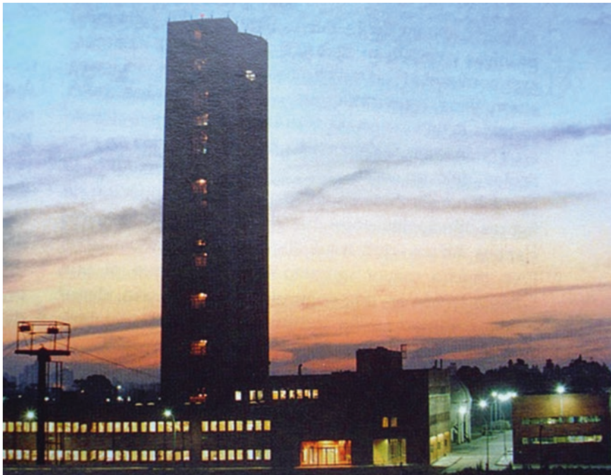
Photo 2.95 The tower of Constituyentes is emblematic and “watches over” the site
