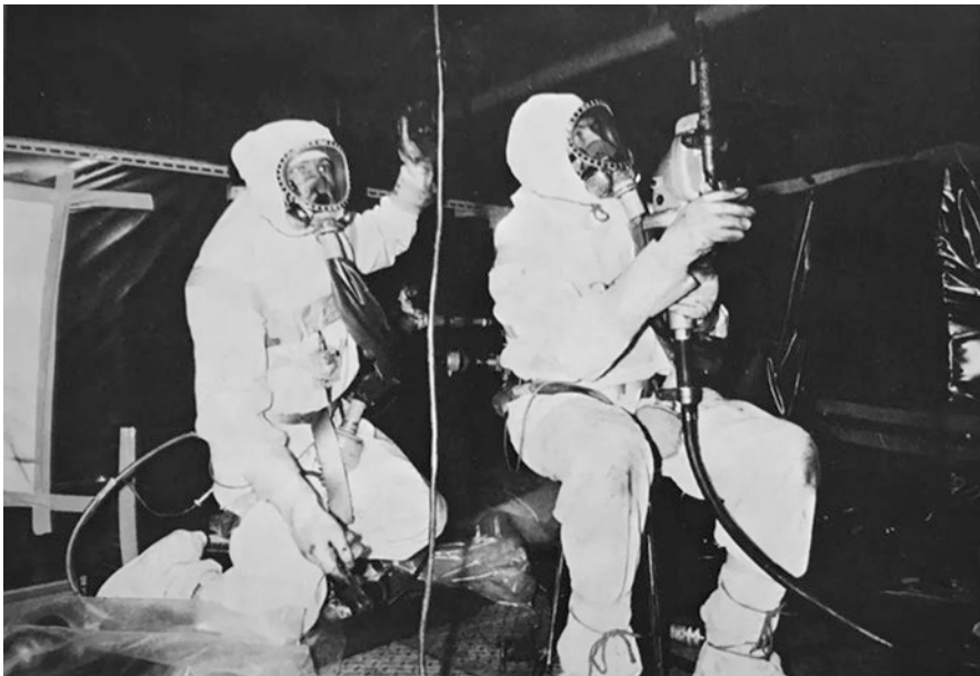
Photo 2.87 Cutting operation on Saint Laurent-A1 during post-accident repair. The operators are wearing ventilated clothing indicating a possible source of contamination
