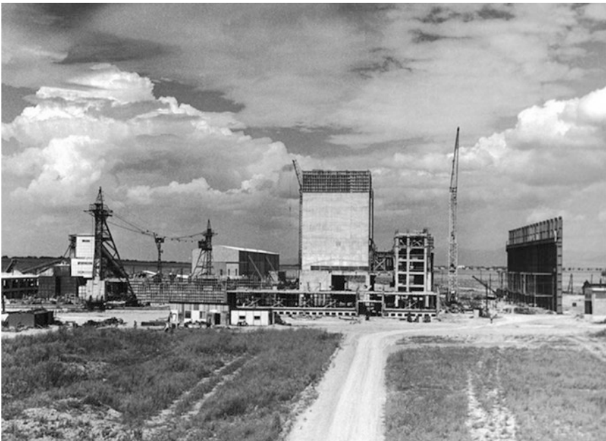
Photo 2.89 Beginning of the A1 reactor construction (circa 1959)
