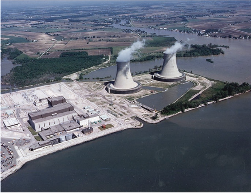
Photo 2.41 The Fermi-2 air coolers. The Fermi 2 reactor is a 1170 MWe boiling water reactor (BWR), commissioned in 1985, initially for 40 years (2025) and built by General Electric which is owned by DTE Energy and operated by its subsidiary Detroit Edison
