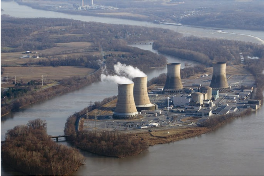
Photo 3.3 Unit-1 in operation. Two cooling towers are required to cool the condenser. The auxiliary cold source comes from the river
