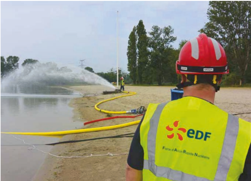
Photo 5.19 Fresh water pumping test by FARN (Bugey). Taps were placed in 2013 to be able to re-supply the backup circuits with water
