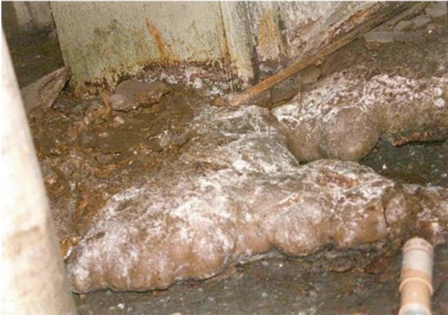
Photo 4.11 Flow of solidified corium in the shape of an “elephant’s foot.” Even after partial solidification, the residual power can melt this corium until the surface in contact with the air is large enough to evacuate the power by natural convection. The activity of this corium is such that the remotely operated inspection robots that approached it the first time failed due to the intense radiation (photo DR)
