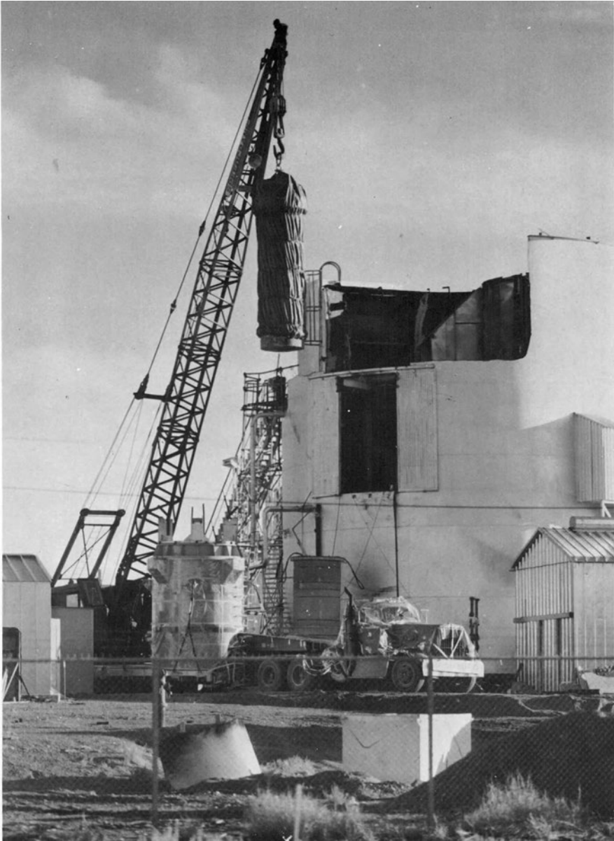
Photo 2.35 Extraction of the vessel through the reactor dome with a mobile crane. A trailer truck carries a transport cask for the vessel
