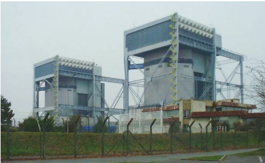
Photo 2.79 The two reactor blocks of Saint-Laurent-A1 and A2. The welded structures that surround them are characteristic of the French Natural Uranium-Graphite-Gas (UNGG) of the late 1960s
