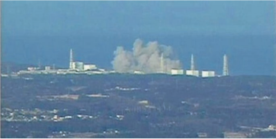
Photo 5.7 A picture of the explosion of reactor-1 taken on TV (NHK). On the left, reactors -5 and -6 and their shared chimney. On the right, reactors -2, -3, and -4 whose buildings are still intact
