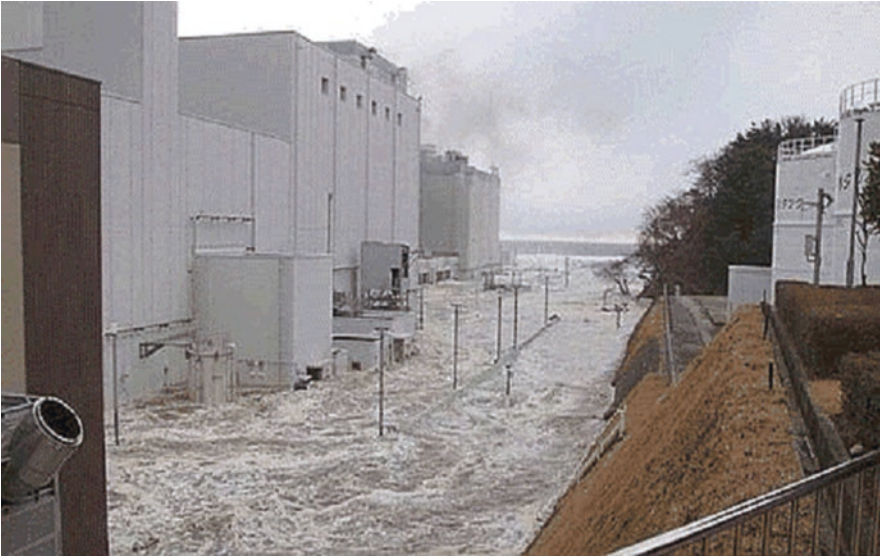
Photo 5.2 Fukushima plant drowned by tsunami—March 11, 2011 (photo Tepco)
