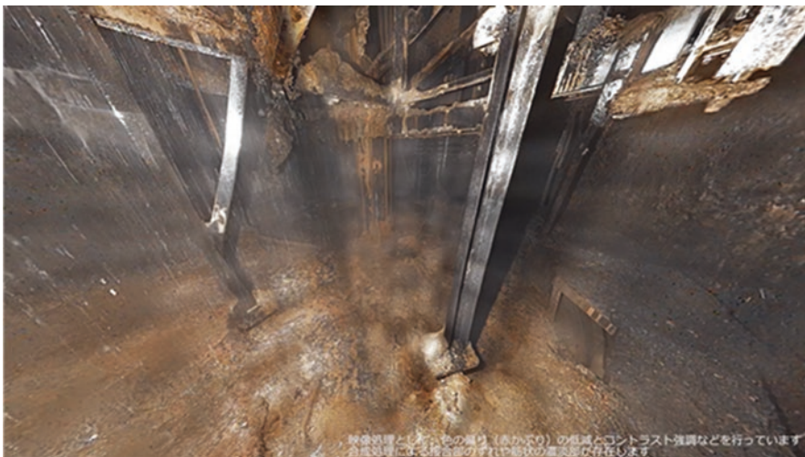
Photo 5.16 Reactor-2 vessel pit. One can see the vessel bottom torn open by the molten corium and the solidified corium, which has spread in the dry pit (photo TEPCO). One should be wary of the pasty aspect that the cooled corium takes because a metallic corium in meltdown can be more fluid than water
