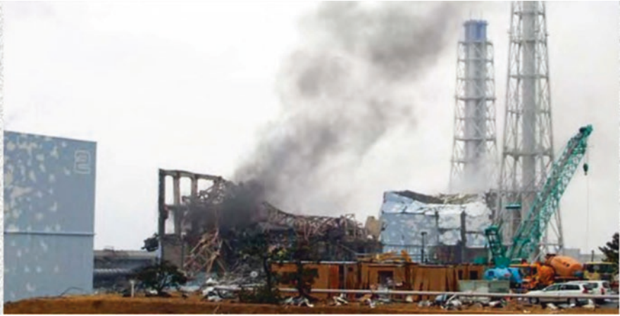
Photo 5.6 Reactor-3: The disturbingly persistent black smoke from Reactor 3 probably indicates an ongoing corium-concrete interaction in the bottom of the dry pit and possibly on the building foundation (TEPCO photo)
