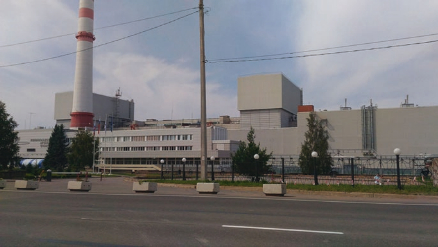
Photo 4.19 Two reactors of Leningrad (the highest cubic blocks contain one reactor each)
