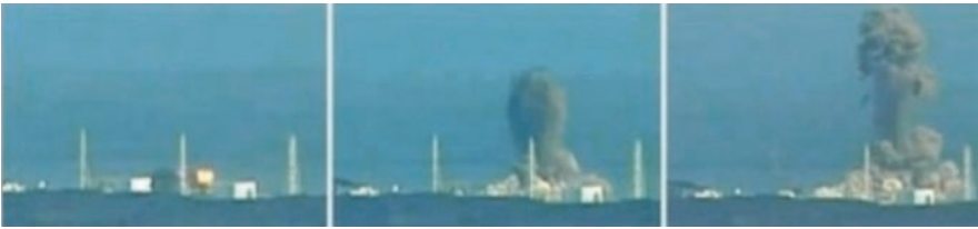
Photo 5.8 Hydrogen explosion in the building of reactor-3 taken on television (NHK). On the left reactor-2, on the right reactor-4
