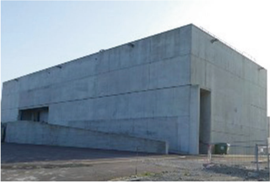
Photo 5.18 The first Local Crisis Center in Flamanville (France) went into service on January 10, 2020, the site that will host the first French EPR. The strongly defended and particularly austere building (blockhouse without windows!) contains 2500 m 2 of premises. It has 72 h of electrical autonomy and has three floors located more than 20 m above sea level to avoid submergence. The means of communication have been particularly studied. This unique building, built in 5 years, allows 3 days of autonomy to the teams who would use it. All French nuclear sites will progressively be equipped with a Local Crisis Center (photo EDF)
