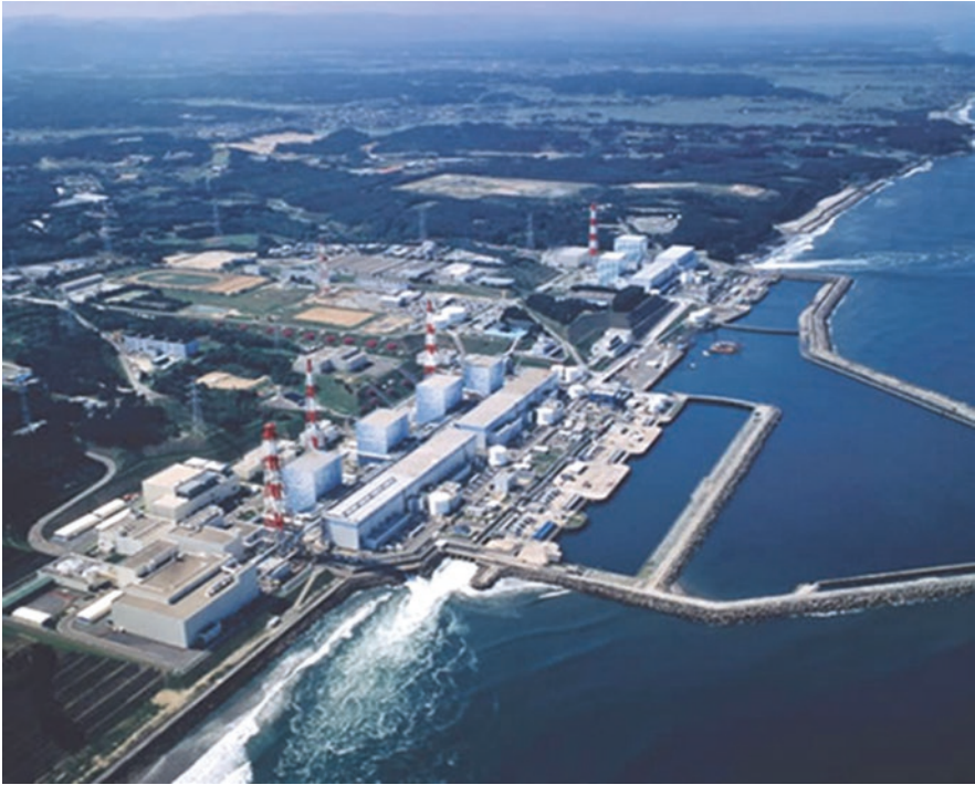
Photo 5.1 The Fukushima Dai-ichi plant: in the foreground, unit 4 appears as a cube located between the two red and white towers, then reactors 3, 2, and finally 1 (Photo Tepco). A large gap separates Reactor-1 and Reactors-5 and -6 sharing a ventilation stack painted in white and red. The building located between reactor-1 and reactor-5 along the coast is the Dry Cask Storage Facility common to all reactors
