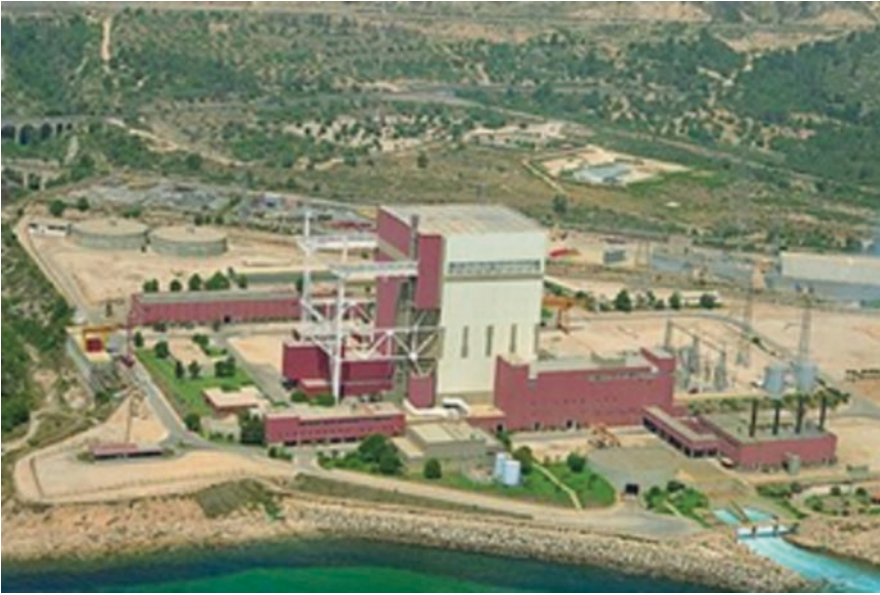
Photo 2.7 The Vandellós-1 plant in Spain
