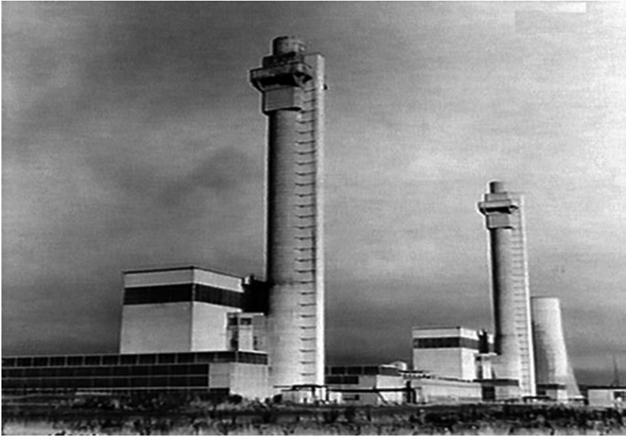
Photo 2.1 An ominous-looking photo (cloudy sky? low angle shot?) of the two military reactors at Windscale. One notices the filters placed abnormally at the top of the chimneys
