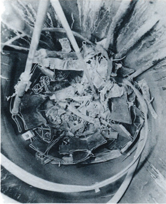
Photo 2.33 View of the core during disassembly (1962, INEL)
