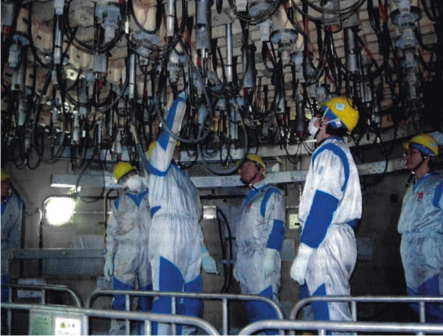
Photo 5.4 Operators inspecting vessel bottom penetrations by control rods on a Fukushima Dai-ichi plant. The reactor core, shutdown in this photo because one does not go into the reactor pit during operation, is thus located above the operators. The system is identical on Fukushima Dai-ichi (TEPCO)
