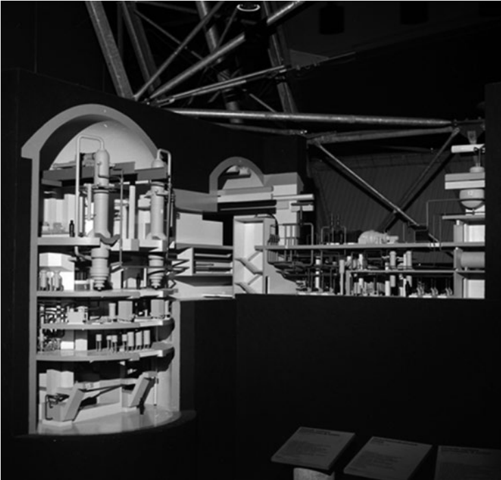
Photo 2.63 Model of the reactor cavern and the turbine cavern. One recognizes well above the reactor the two vertical steam generators of great height
