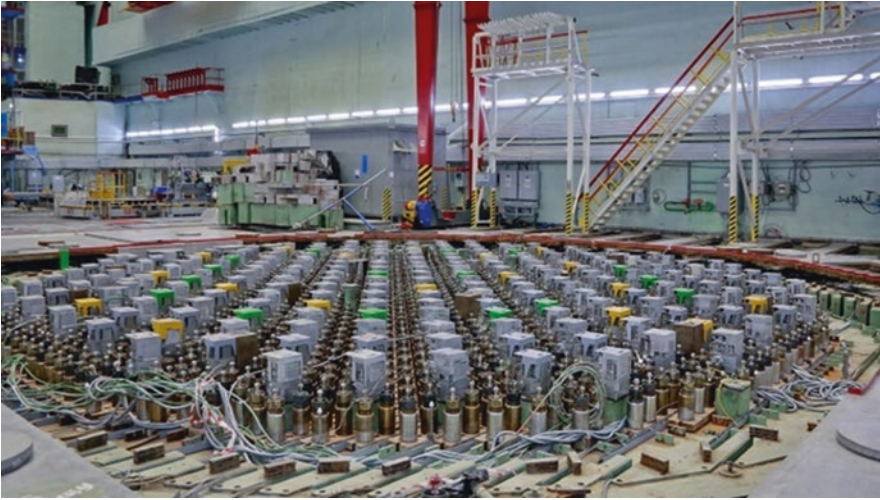
Photo 4.2 Smolensk-3 loading face being upgraded (photo Rosatom)
