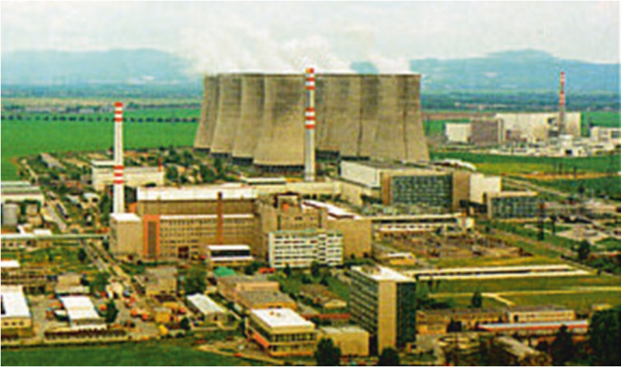
Photo 2.90 The site of Bohunice. The A1 reactor is recognizable with its very high hall with white roof and by the chimney on its left. The eight air coolers in operation serve the 4 WWER-440 reactors on the right of the picture
