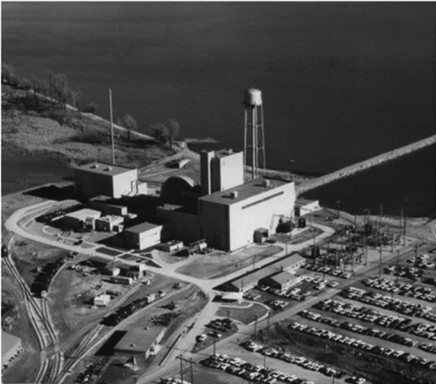
Photo 2.39 Fermi-1 plant in the sixties
