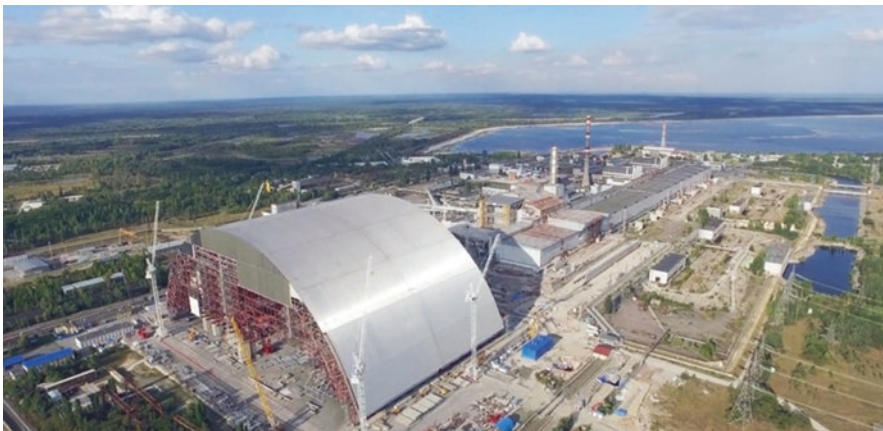
Photo 4.14 The new containment arch built by the French companies Bouygues and Vinci (source site internet Bouygues)
