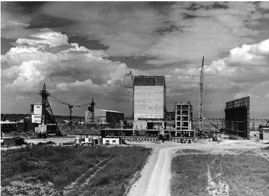
Photo 2.89 Beginning of the A1 reactor construction (circa 1959)
