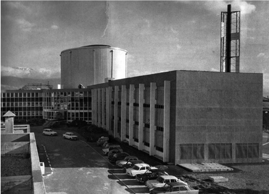
Photo 2.52 Siloé building inside the CEA site. The reactor is located in the white cylindrical building
