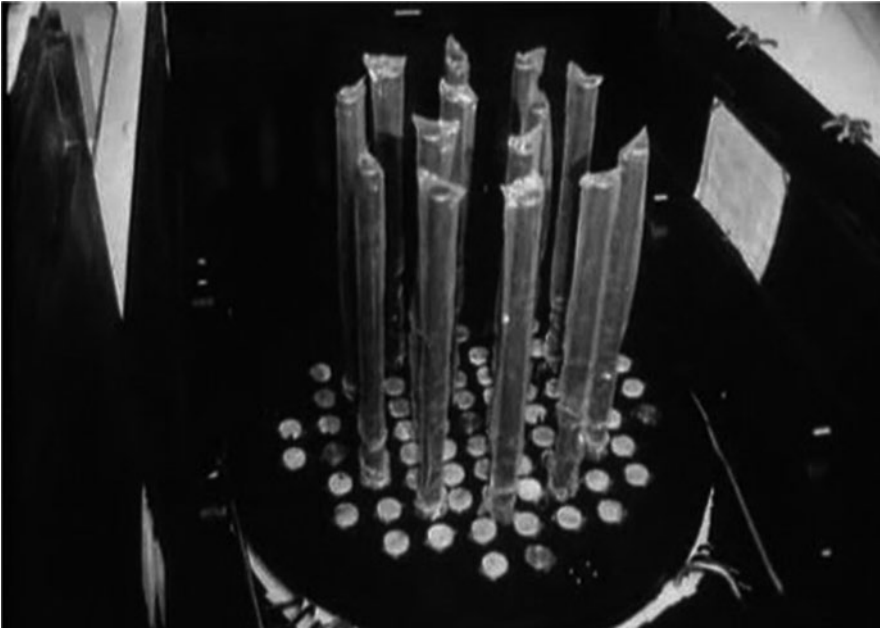
Photo 2.67 View of the upper side of the Lucens reactor vessel (photo IFSN). The control rods and shutdown control rods, wrapped in transparent plastic, can be seen emerging from the vessel cover
