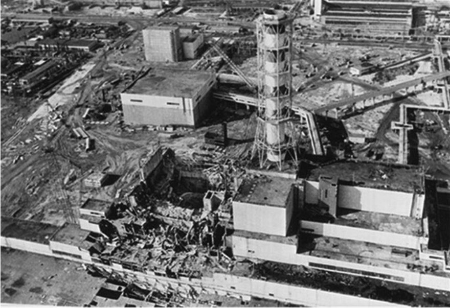
Photo 4.9 Aerial view of the reactor-4 or rather what remains of it. This view allows to see inside the pit of the reactor
