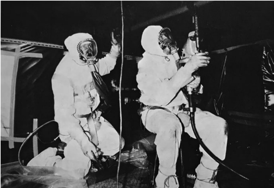
Photo 2.87 Cutting operation on Saint Laurent-A1 during post-accident repair. The operators are wearing ventilated clothing indicating a possible source of contamination
