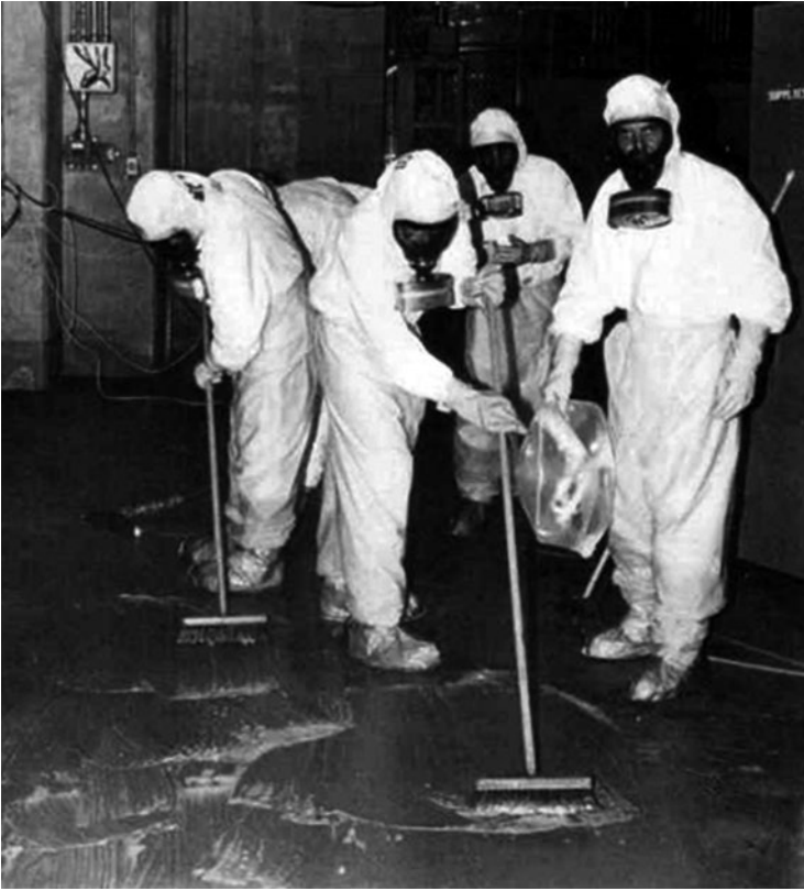
Photo 3.6 Cleaning the floor for decontamination
