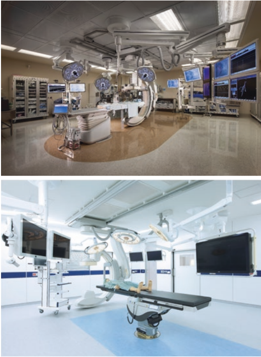
Fig. 3 Two types of “hybrid” suite with imaging compatible table, mobile fluoroscopic C-arm, large monitors, and anesthesia machine. (Note: Cardiopulmonary bypass unit is not pictured, but should be readily available)
