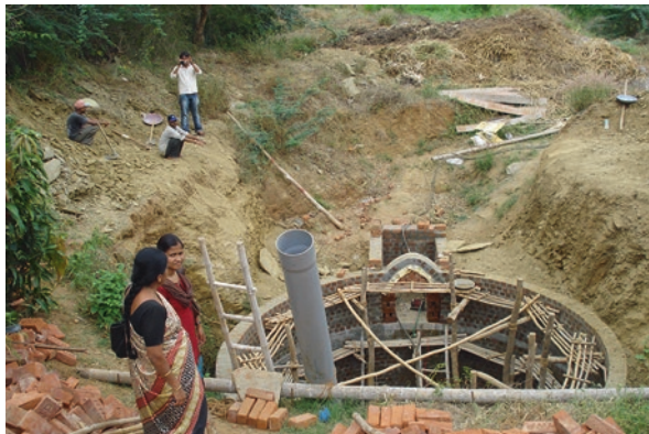
Fig. 3 View of installation of 45-m 3 solid-state biogas plant at Airani Ashram
