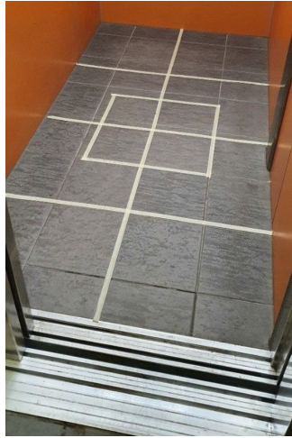
Fig. 3. Marking of the elevator floor area into sections of the location analysis model.
