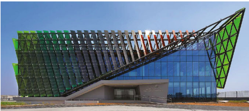
Fig. 8.2 Amorphous silicon vertical fins—double skin, DEWA Research center, Dubai, UAE (courtesy of Onyx Solar)
