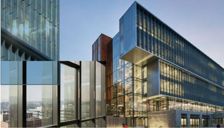
Fig. 8.1 Amorphous silicon vertical fins—Life Science Building, University of Washington, Seattle, USA (courtesy of Onyx Solar)
