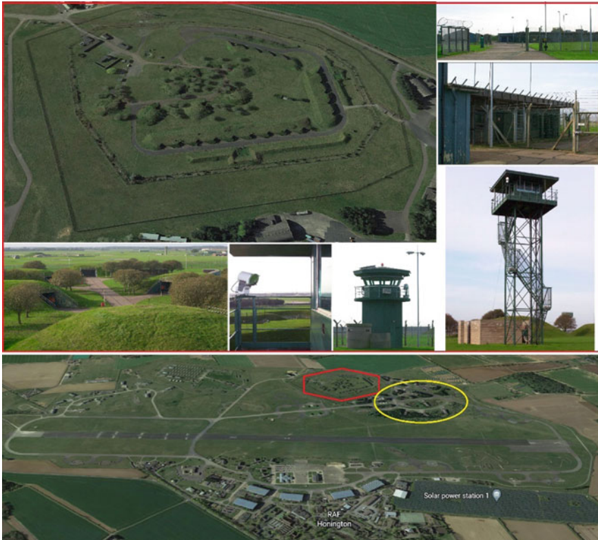
Fig. 5 Special weapons storage facility
