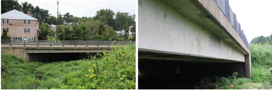
Fig. 2 Foulk Road bridge in Wilmington, DE
