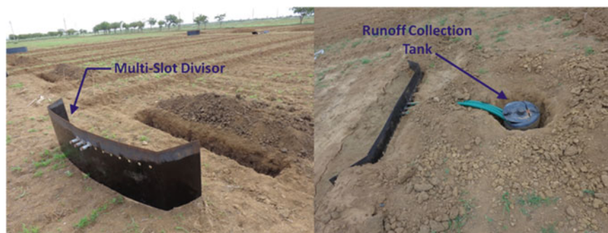
Fig. 8.4 Installation of fabricated multi-slot divisor and runoff sampling tank
