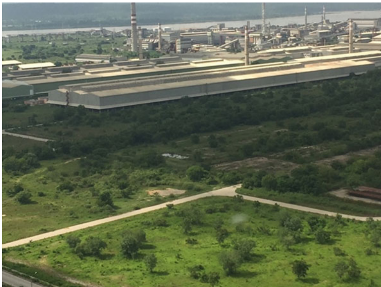
Fig. 5 Ajaokuta Steel Plant, Zombie of Nigerian Steel Ambitions, in the Summer of 2019 (photo by the authors)
