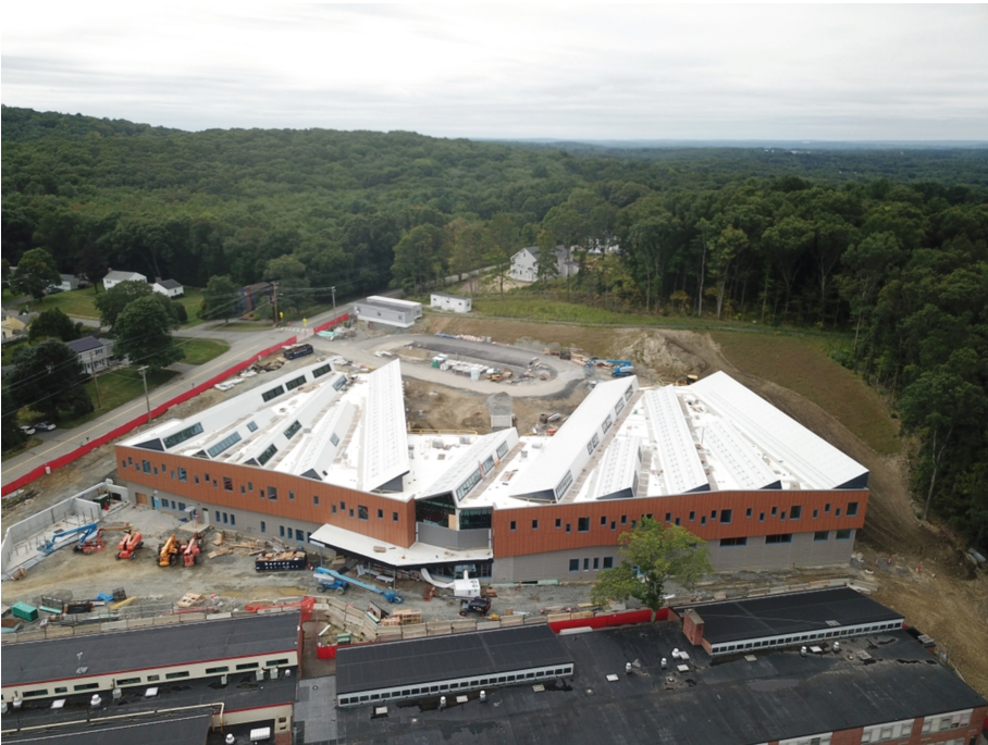
Fig. 15. Fales Elementary School during construction with existing school in foreground
