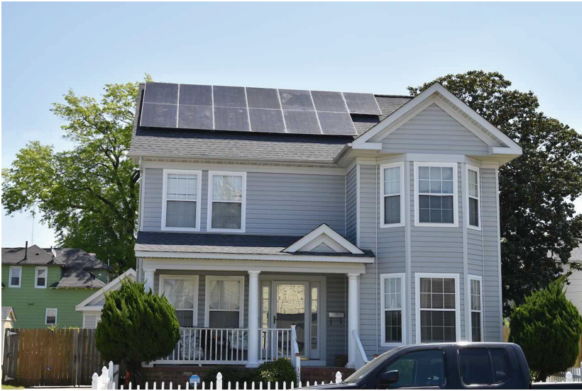
Fig. 2. The first residence in Virginia with solar installed via a PPA.
