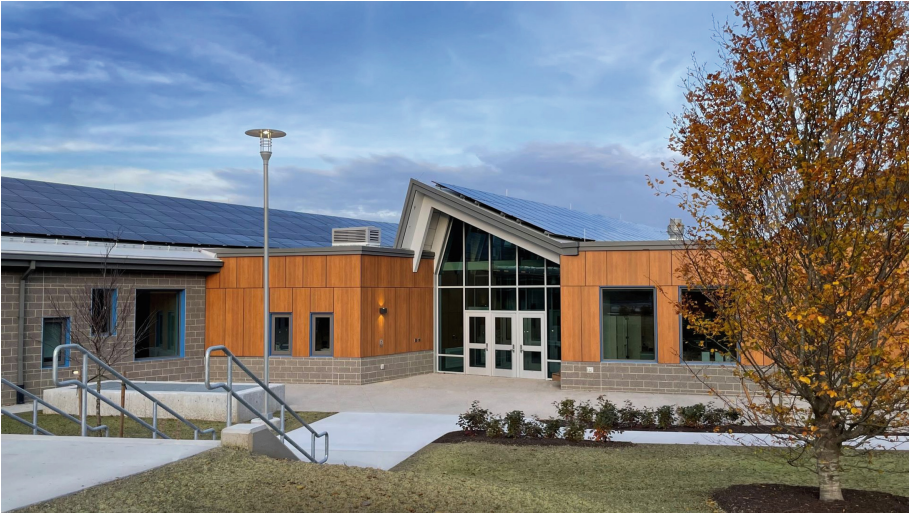
Fig. 16. Annie E. Fales Elementary School main entrance
