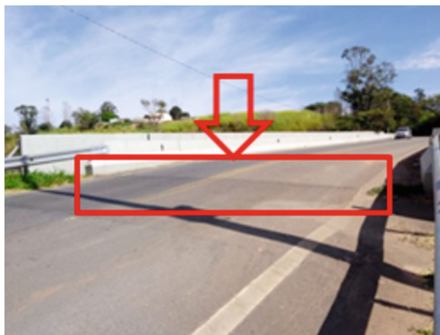
Fig. 5. Manoel Aveiro viaduct (Color figure online)
