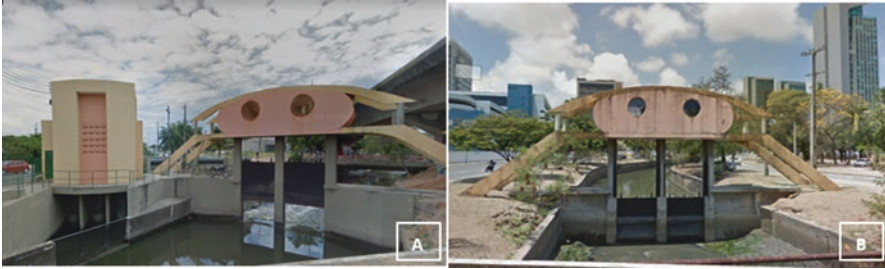
Fig. 14.3 Gate system (a) gate and pumping station at the north end. (b) Gate at the south end. (Source: authors)
