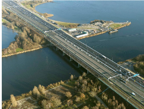
Fig. 1. The Hollandse Brug bridge [11]
