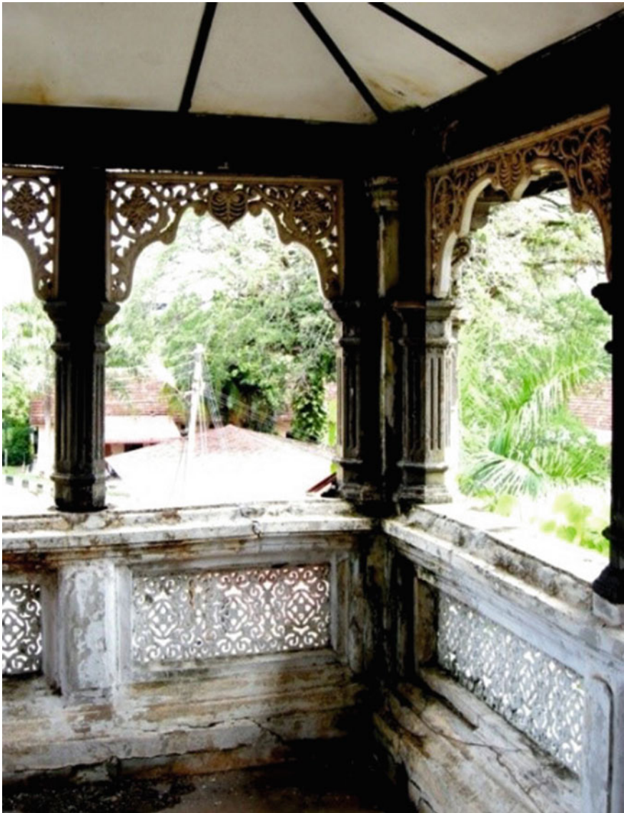
Fig. 6 The balcony on the second floor
