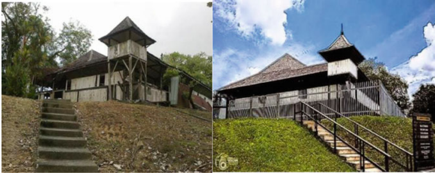
Fig. 4 Alice pillbox in Sarawak before and after conservation work Source Mai Singgah (2018) (Right) and Tengku Halbert (2018) (Left)
