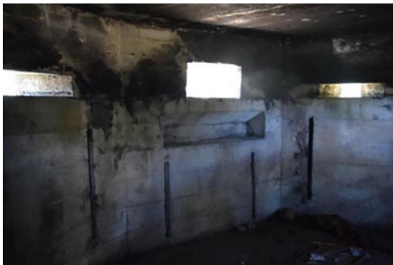
Fig. 2 Wall structure inside British pillbox in Kelantan Source Field study
