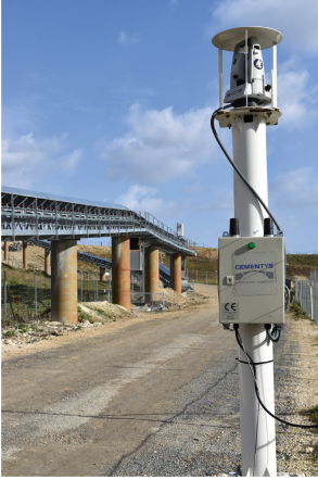
Fig. 3. Conveyor belt & Robotic Total Station
