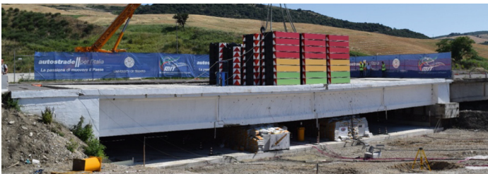
Fig. 4. Pictures of the Alveo Vecchio viaduct during the P5 phase
