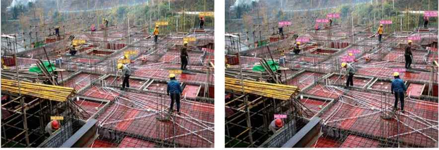
(a) Detection results of traditional YOLO v5s algorithm (b) Detection results of improved YOLO v5s algorithm
