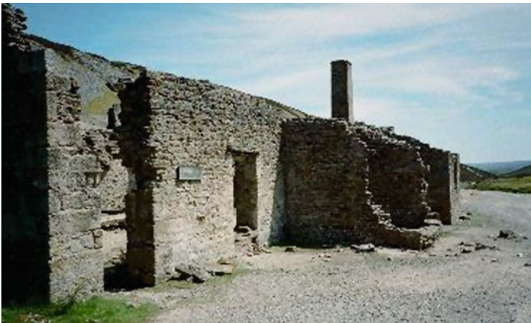
Fig. 25.11 Remains of the Old Gang Smelt Mill. Photo by the author
