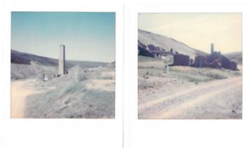
Fig. 25.13 Chimney still stands within the ruins of the Smelt Mill at Old Gang Mines. This is because many stones have been reclaimed to build in other places over time. Photo by the author
