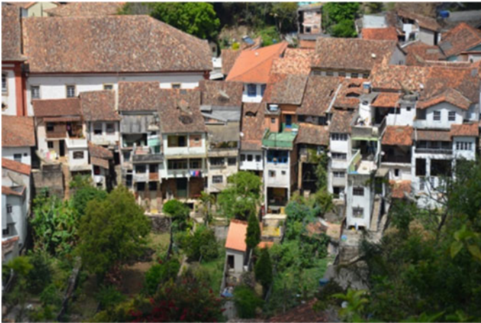
Fig. 4.5 View of the rear of some houses
