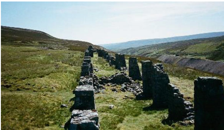
Fig. 25.10 Remaining structure of the Smelt Mill storage barn shows the large stone pillars, approximately 1 m in depth. Photo by the author
