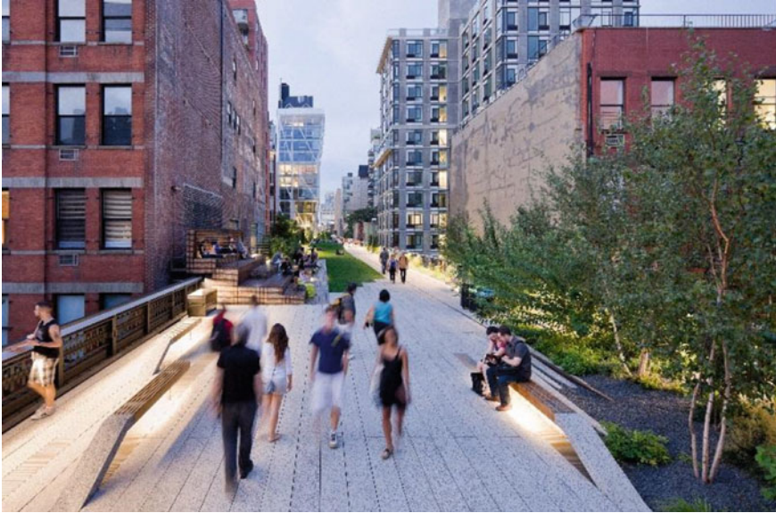
Fig. 14.14 Highline walkway, US. Arch. Diller Scofidio + Renfro, J. Corner, P. Oudolf. Source Courtesy of Diller + Scofidio
