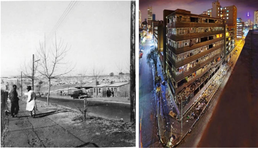
Fig. 10.1 Left: Orlando was one of the first black townships established as part of the relocation policy in 1960 Chipkin, Clive (1993). Right: Hijacked buildings in Hillbrow. Photo credit L. Krige
