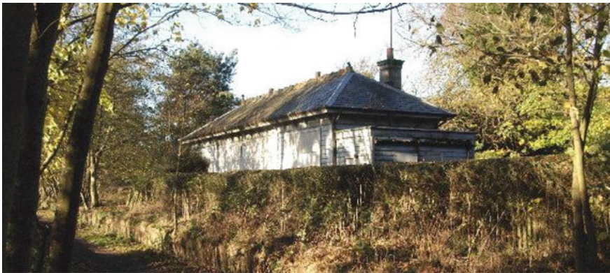
Fig. 14.8 Pitfodels station before the restoration, Aberdeen. Source P. Ward geograph.org.uk
