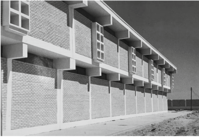
Fig. 5.9 Lack of exterior glazing shows that Roth designed it for the Gulf climate; however, the forms and proportions are reminiscent of his European work ( Source gta Archiv, ETH Zurich)
