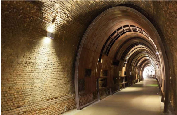
Fig. 14.12 Albisola tunnel, Italy. Arch. 3S Studio. Source Courtesy of 3S Studio
