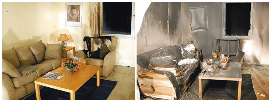
Fig. 11.1 The performance of a residential sprinkler (left) with limited fire damage as compared to the fire damage caused by flashover (right). (Photos from the video “Residential sprinkler saves lives” from 2001 [14])
