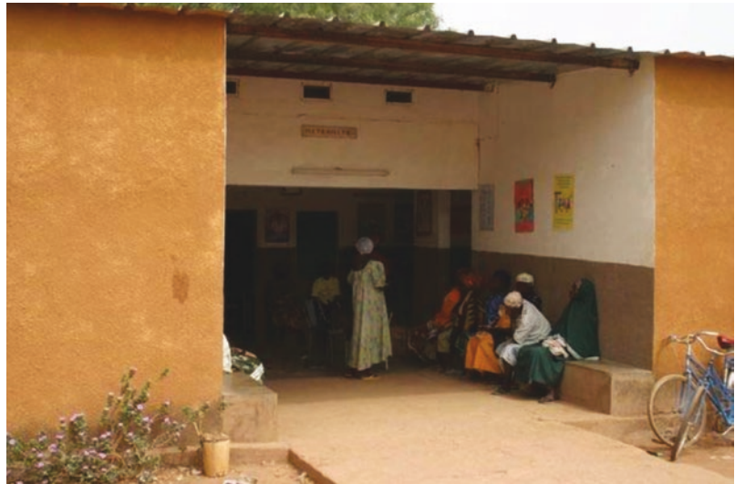
Fig. 25.1 Maternity unit of the Medical Centre with Surgical Services [Centre Médical avec une Antenne Chirurgicale (CMA)] that serves most women in Boromo health district. (Photo Credit: Aduragbemi Banke-Thomas)
