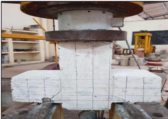
Fig. 10.4 Failure pattern for corbel without shear reinforcement
