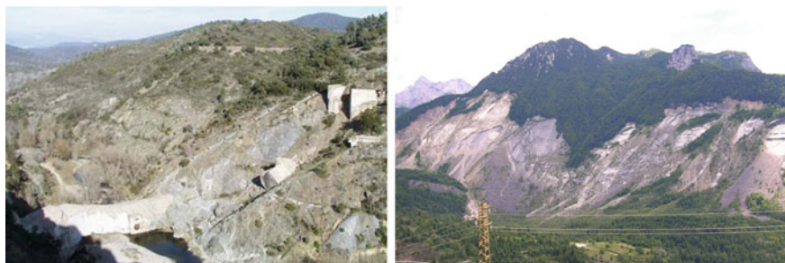
Fig. 1 Malpasset dam failure ( left ), and Mont Toc (Vajont) landslide ( right )
