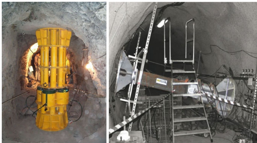
Fig. 19 Plate loading tests in an adit ( left ) [45], and in a tunnel ( right ) [46]
