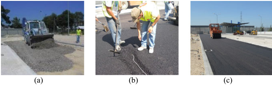
Fig. 8 Instrumentation and construction of the full-scale experimental sections [32]
