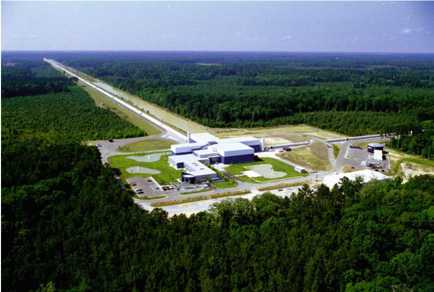
Fig. 3 Aerial view of LIGO-Livingston site (Credits The LIGO Collaboration) https://www.ligo.caltech.edu/system/avm_image_sqli/binaries/30/jpg_original/ligo-livingston-aerial-02.jpg?1447107179
