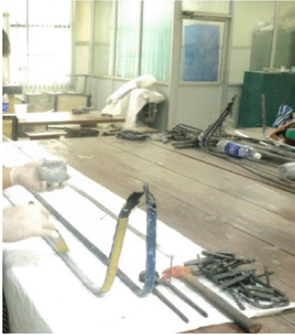
Fig. 2. Using a brush to apply The Sikadur®-330.
