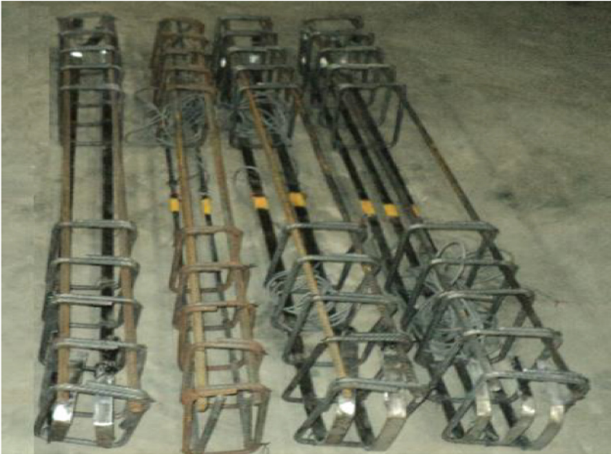
Fig. 4. Reinforcement cages of beams.
