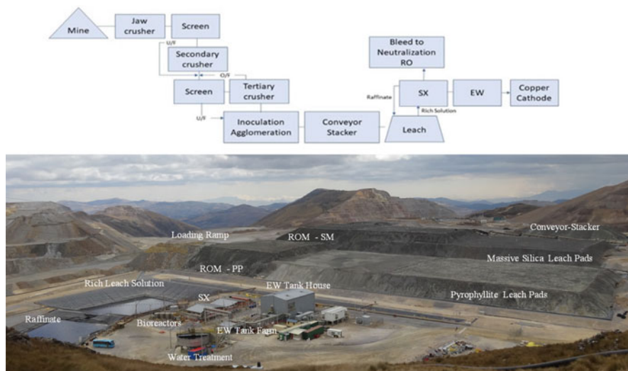
Fig. 10.1. Flowsheet for the enargite bioleach and actual layout of the bioleach demonstration facility at Yanacocha
