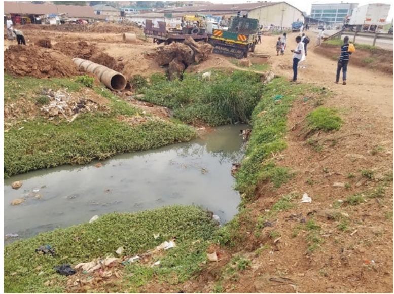
Fig. 18.10 Rubbish dumps are situated very close to the drainage canals, and some are evidently blocked, leading to stagnant water
