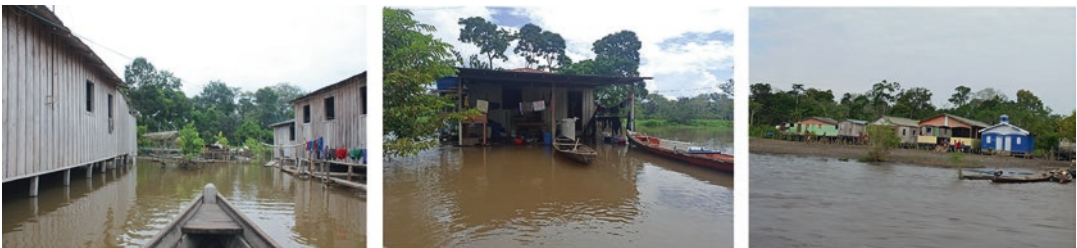
Fig. 25.2 Examples of buildings in riparian communities are characterized by proximity to water
