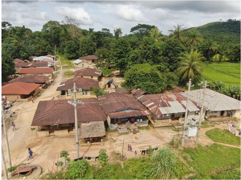
Fig. 11.3 A drone image of Lunsar, Sierra Leone provides a glimpse of how the power grid does not reach everyone
