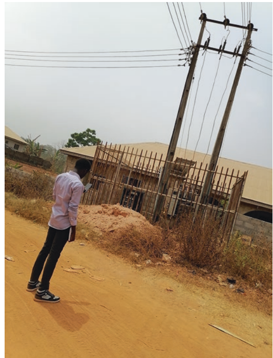
Fig. 12.6 Transmission lines are important features that require field mapping or validation
