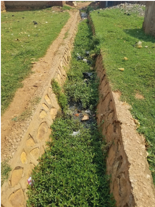
Fig. 18.8 Some drainage canals like this one in Kalerwe are fully covered by vegetation
