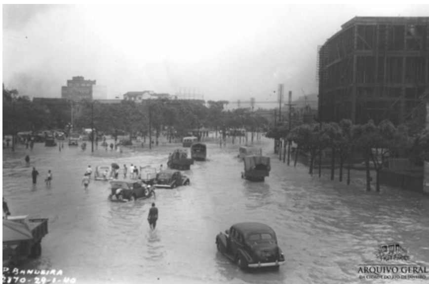
Fig. 3 Photograph of Praça da Bandeira, in 1940, showing the occurrence of floods that periodically reach a consisting mangrove embankments area in a confluence of rivers that flowed into the Saco de São Diogo in the past. Source Malta, 29 Jan. (1940)
