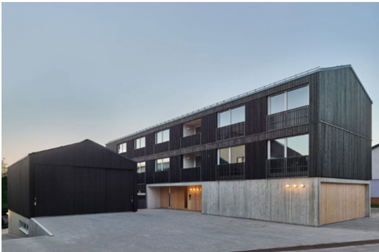
Fig. 14 Schwaikheim housing and workshop (Hinton 2020)
