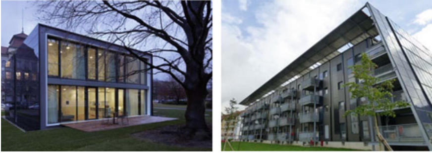
Fig. 12 Two NZEBs visited by CA EPBD: on the left, a single-family demonstration house in Berlin (Germany); on the right, a renovated multifamily house in Graz (Austria) (Hinton 2020)
