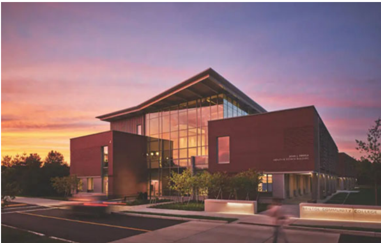
Fig. 16 Bristol Community College's John J. Sbrega health and science building (Hinton 2020)
