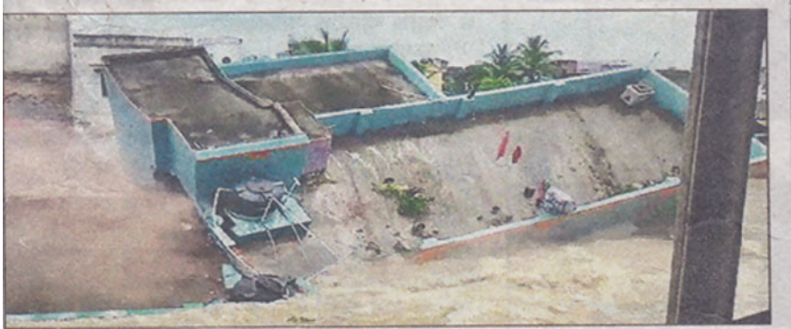
Fig. 4 A two-storied house was washed away due to floods following heavy rainfall in Junbadia village in Bankura district of West Bengal as observed on 6.8.2018
