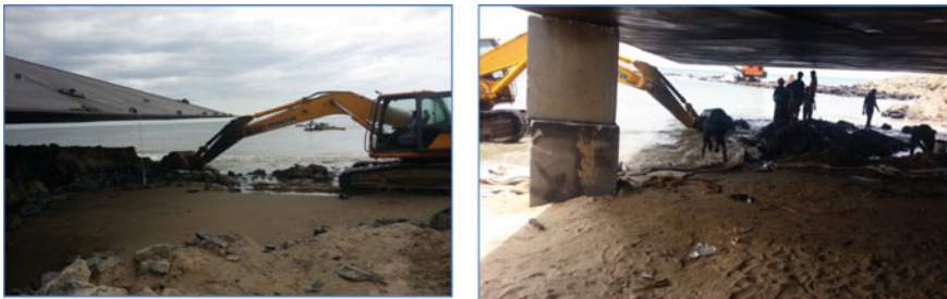
Fig. 1 Base preparation for placing airbags
