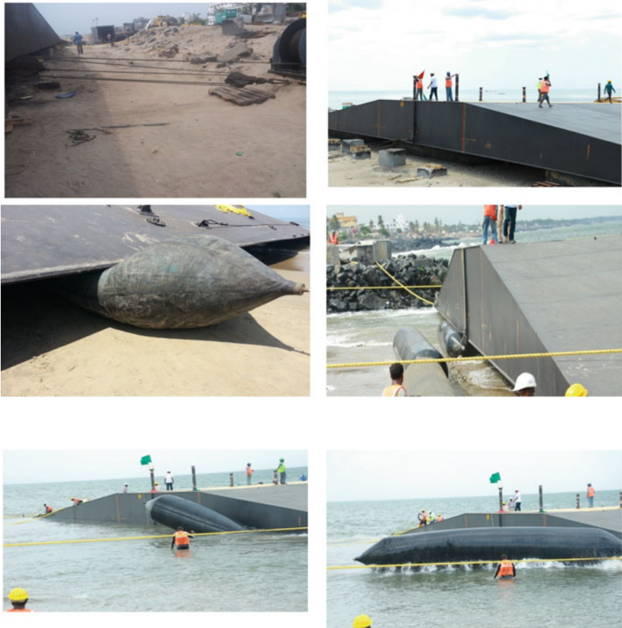
Fig. 5 Stages involved in installation of steel caisson through airbags
