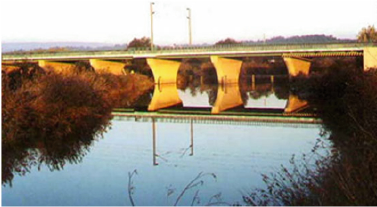
Fig. 5. General view of the Canelas railway bridge (Rocha et al. 2016).
