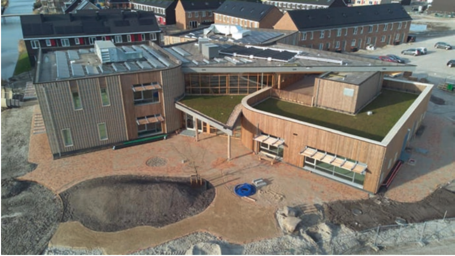
Fig. 19 The green and energy roof of the school with solar thermal collectors and PV panels. [Photo: ORGA architect]
