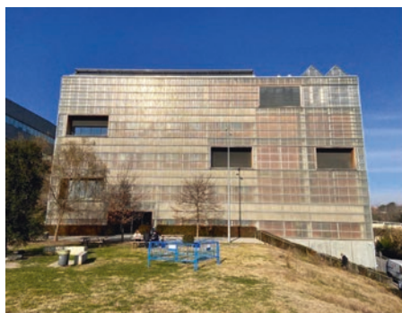
(a) The façade of the ICTA building with shading elements and smart technologies
