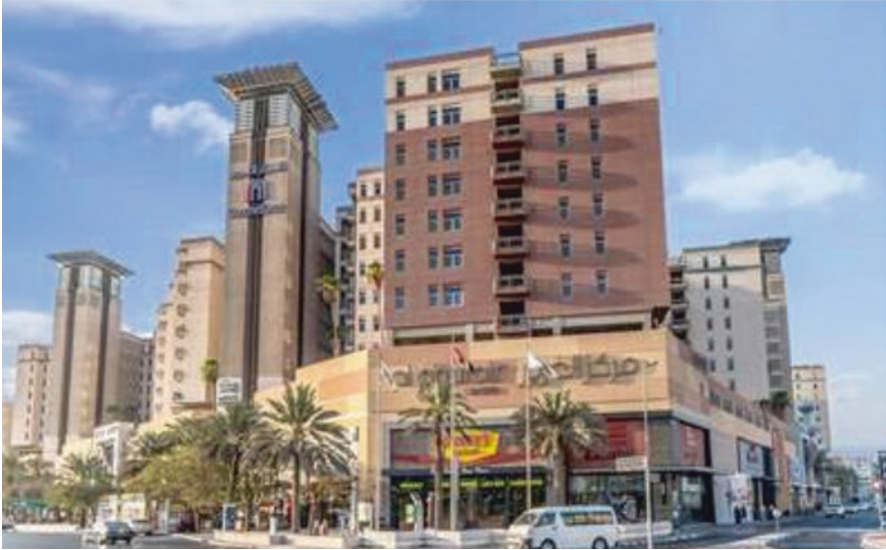
Fig. 13 Al Ghurair Center in the middle of old Dubai, UAE; combining multi-use buildings to rewards the high price of land by using the concept of low-rise high density. Imitating traditional forms like the wind tower to be used as building lifts and landmark as a vertical element. Residential blocks on the left side consist of a large courtyard on third floor where all the amenity activities take place
