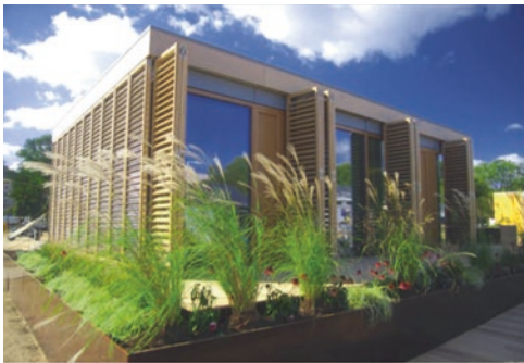
(a) Intelligent facades with integrated photovoltaics on automated wood louvers
