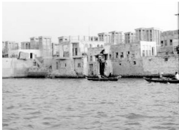
Fig. 2 In Abu Dhabi during the 1940s, several Badgirs or Barajils have demolished with the modernization era of the twentieth centuries
