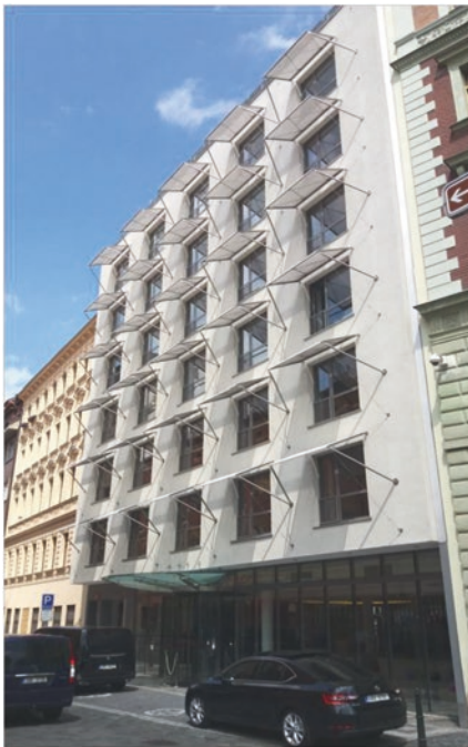
(a) General view of louvers on the main façade
