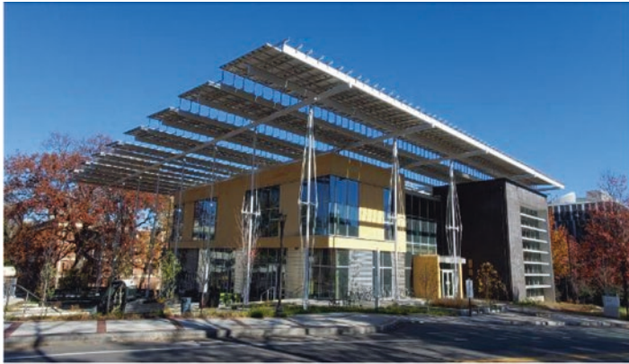
(a) The large roof with integrated Solar PV panels to provide shades on the building's facades
