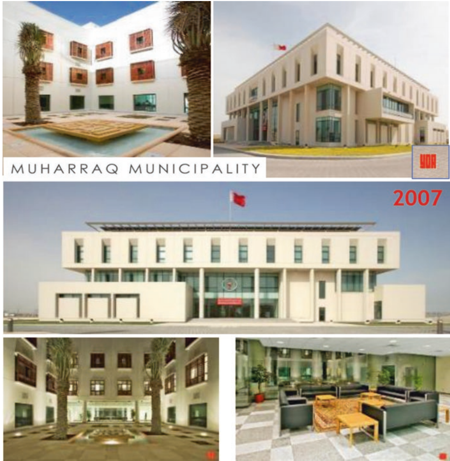
Fig. 19 Muharraq Municipality building in Bahrain (when shaded, a shadow inner courtyard is the key to provide a successful sustainable urban environment). (Source: Youisif Dawood AlSayagh Office, Bahrain 2007)
