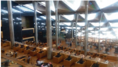
(c) Skylights providing daylight without glare to the readers in the main reading area inside the library
