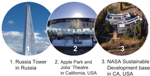
Fig. 20 Examples of examined buildings depicting shading Strategies in Russia and the USA. (Source: Developed by authors)
