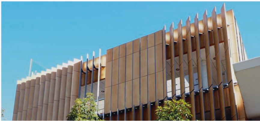
(b) The automated vertical timber louver system to adjust to solar heat, track the daylight ensuring maximum benefit of natural light
