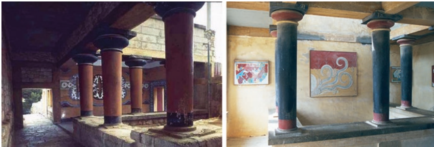
Fig. 8 (Restored) light wells in the Hall of the Royal Guard in Knossos. (Source: K. Tsikaloudaki: "Shedding light on constructions of the past and today: the use of advanced daylight systems through the centuries", international symposium "Advanced Daylighting and Artificial Lighting in Architecture in 21st Century", Seoul, 18.06.2006, proceedings pp. 119–153)
