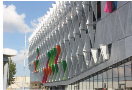
(b) Vertical triangle-shaped shading louvers in the main façade to provide daylight and control glare
