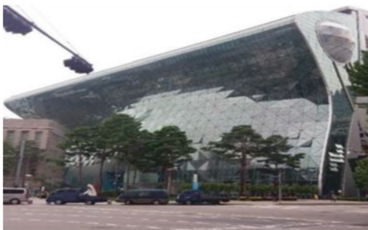
(a) High reflective Low-E glazing facade to reduce heat gain and inclined from the top creating a self-canopy to provide shadow
