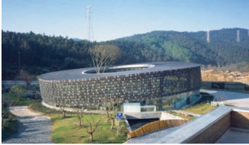
(a) The circular façade with a copper tiles screen controlling daylight into building spaces
