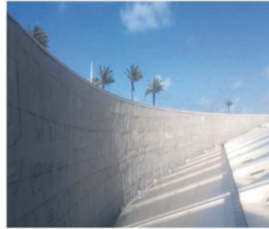
(b) The external curved granite wall provides shading on the inclined roof surface
