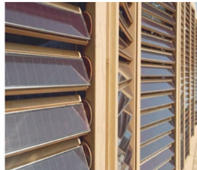
(b) Automated louvers with solar PV to generate energy, regulate heat and daylight
