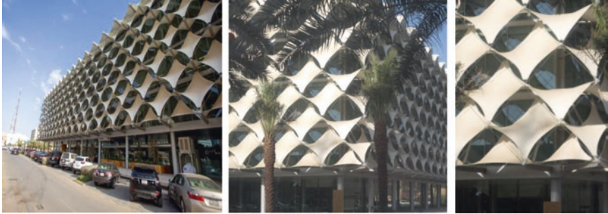
(a) Side view of the library's double-skin lightweight textile façades
