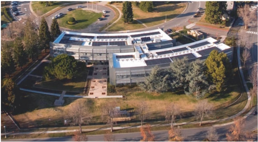
(b) Double-skin façade with external shading louvers connected to sensors for real-time data to control solar heat, provide indoor comfort, and solar panels on roofs
