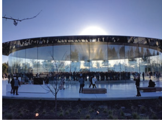
(a) The Cylinder form and cantilever roof provide shades, cooling, and ventilation
