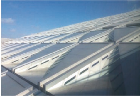
(a) External view of the inclined roof with integrated triangular shaped skylight for daylighting
