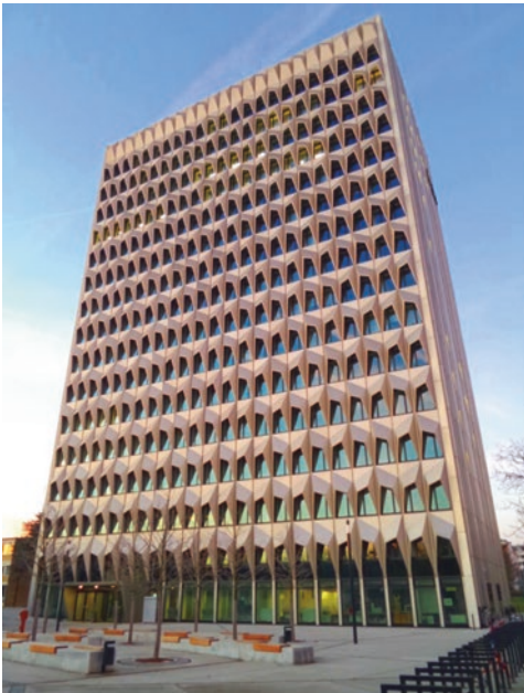
(a) Haus C10 building's with 3-D light metal folding elements as sunshades for widows' balancing light and sun protection
