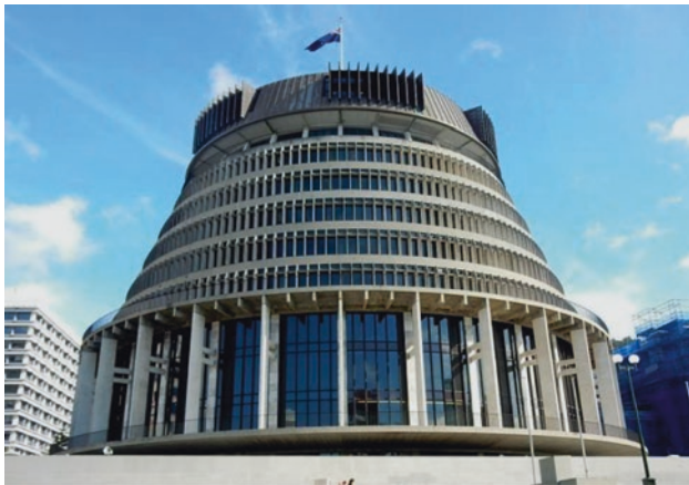
Fig. 16 The Wellington Beehive Parliament Building's conical shape with shading screen in New Zealand. (Image credit and source: Michael Coghlan, https://commons.m.wikimedia.org/wiki/File:The_Beehive_(26564318913).jpg# )
