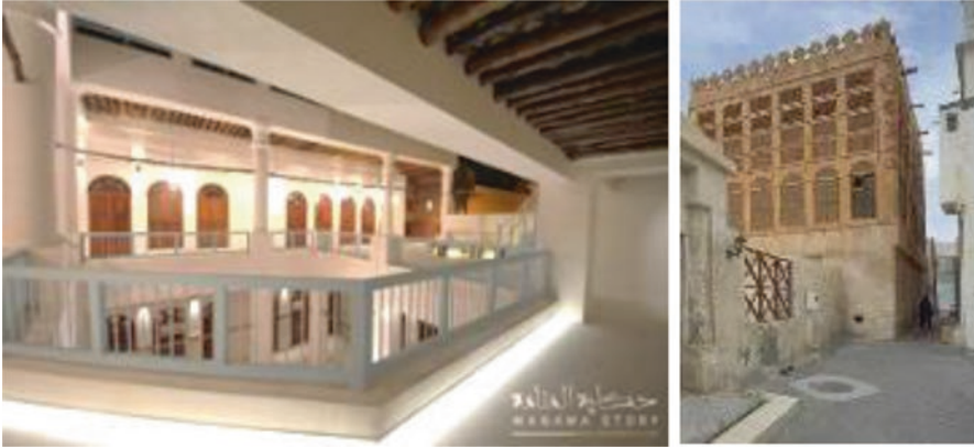
Fig. 8 Right: Siyadi House in the heart of Muharraq old town, one of the best examples of building comfort; all these magnificent screens are from Gypsum and wooden windows. Left: Courtyard inside Khalaf House in Manama
