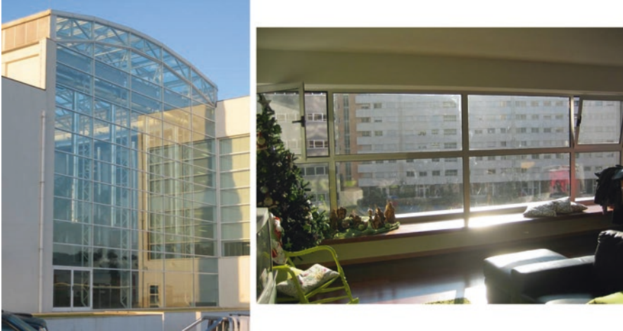
Fig. 1 Constructive solutions that cannot achieve thermal and visual comfort conditions without an excessive and unnecessary energy consumption
