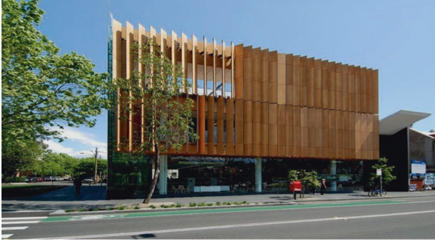
(a) General view of Surry Hills Library and Community Centre in Sydney, Australia
