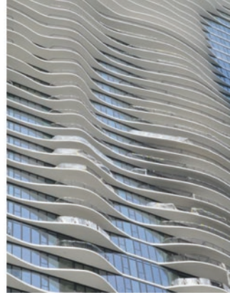
(b) Shading louvers in the façade of the Aqua Tower
