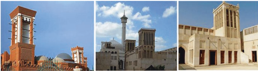
Fig. 5 Different traditional windcatchers in Arabian countries. Windcatchers function during daytime and nighttime. Left: decorative Barjeel in Qatar; Middle: Barjeel in the Bastakiya Quarter of Dubai-UAE; Right: an example of Windcatcher in Bahrain
