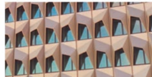
(c) Close up view of the 3-D light metal folding elements to allow for daylighting
