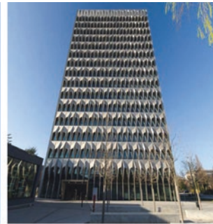
(b) The insulated façade with operable widows for natural ventilation and Brise Soleil for sun protection
