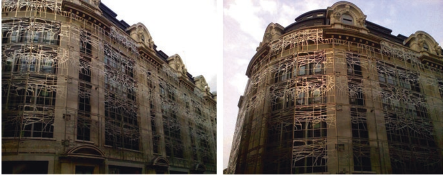
(a) A metallic screen on the façade to provide shading on windows
