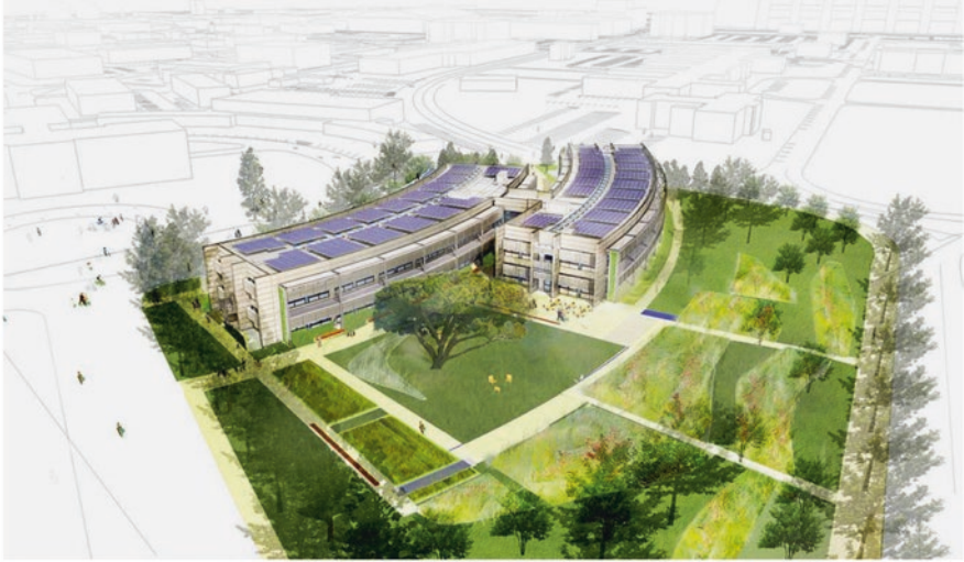
(a) Bird's-eye view of the twin buildings with a space in between to channel air and solar PV panels on roofs to generate electrical energy
