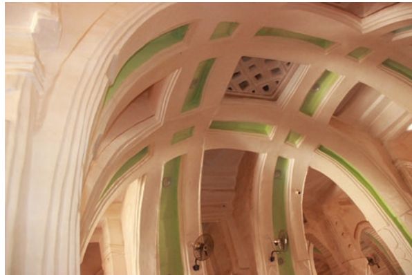
Fig. 5 Zaria mosque columns with mai bakin rijiya (well opening) roofing
