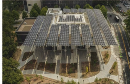
(c) The dynamic roof acting as a chimney to cool the interiors via stack effect and the 330 kW (DC) roof comprising of 917 solar PV panels
