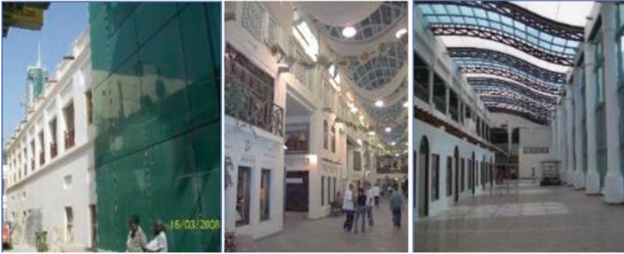
Fig. 20 Development of the new Souq in the traditional town of Manama-Bahrain; using extensive skylight of steel glazed ceiling, increase the heat load and energy consumption with no care of sustainable environment building comfort (2006). This should be not acceptable with the increase of power consumption
