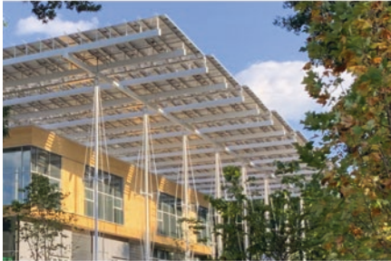
(b) The solar PV canopy providing shading on the building's western façade
