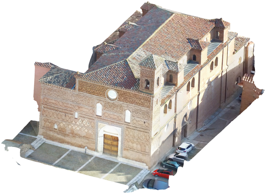
Fig. 3. Axonometric view of the photogrammetric model of Sta. María de Tobed (Prepared by the authors).
