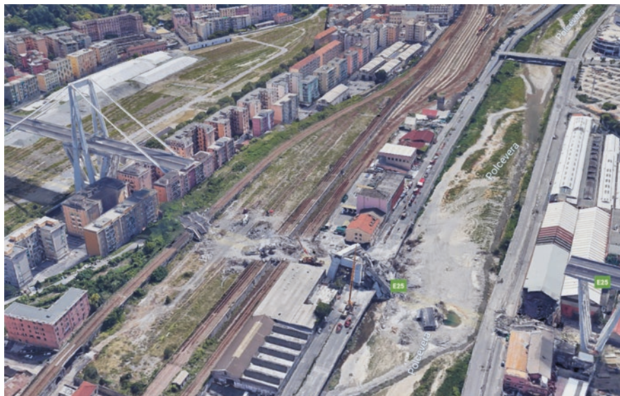
Fig. 3 Collapsed section (Author's elaboration. Source: Google Earth)
