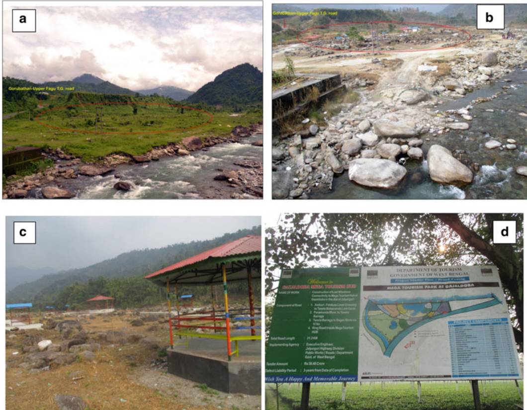
Fig. 2.25 Vacant right lower terrace of Chel River just upstream of Mukti Bridge, Odlabari (Photograph 08.08.2012) (a); amenities for tourists and picnickers developed on the same site (13.01.2016) (b); close up photograph showing various amenities developed for tourists and picnickers on the same site (13.01.2016) (c);
