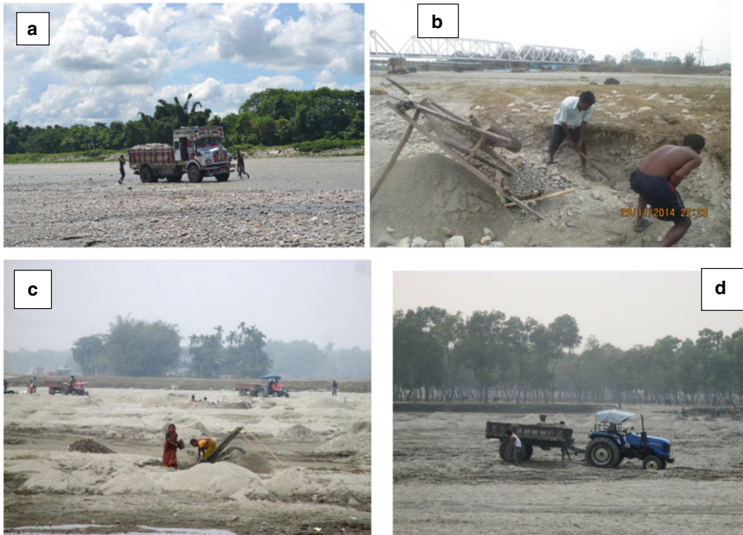
Fig. 2.3 Field photographs showing Boulder lifting at Toribari, Upper Reach (a); mid-channel gravel bar skimming at Odlabari, Middle Reach (b); sand mining at Rajadanga, Lower Reach (c, d)
