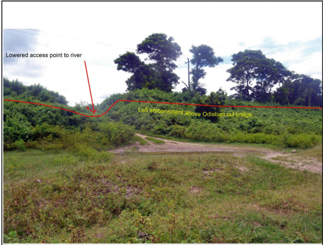
Fig. 2.10 One of the many humans breached embankment points for easy access of men and vehicles into the river
