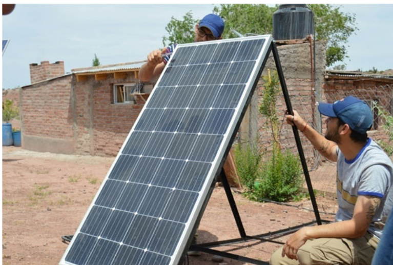
Image 10.3 Final installation of support. (Source: Authors' own work)
