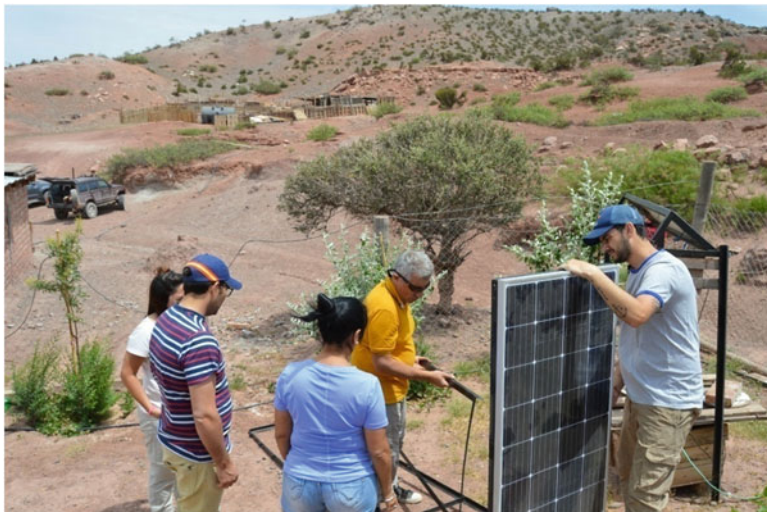
Image 10.2 Final installation of panel. (Source: Authors' own work)
