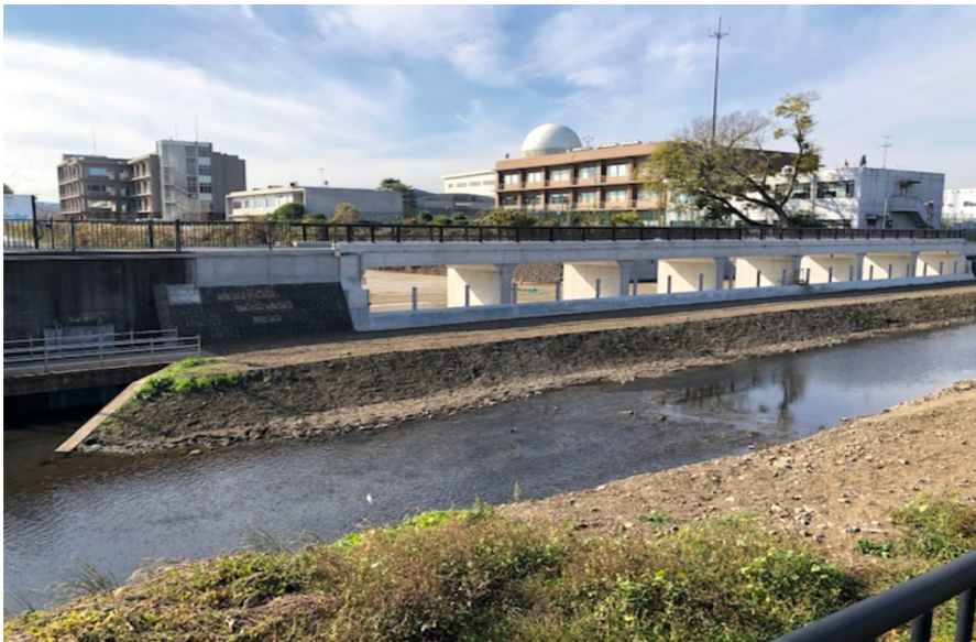
Fig. 10. Rainwater shelter storage pond under expanding construction
