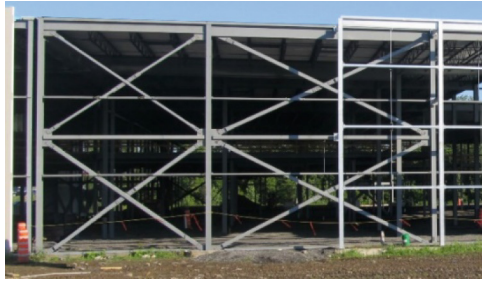
Fig. 1. Example of a two-bay two-tiered CBF.
