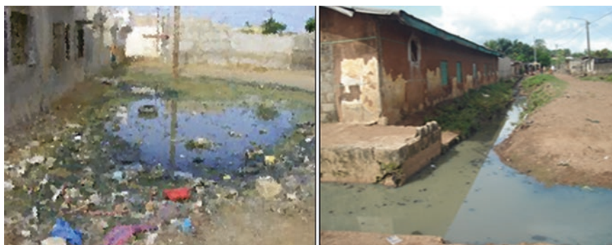
Fig. 1.1 Discharge of wastewater in some rural areas of Morocco.
