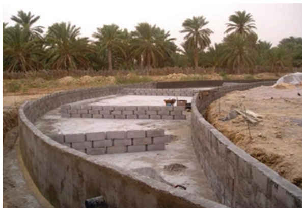
Fig. 2.5 Early construction phase of the constructed wetland at Témacine [55]
