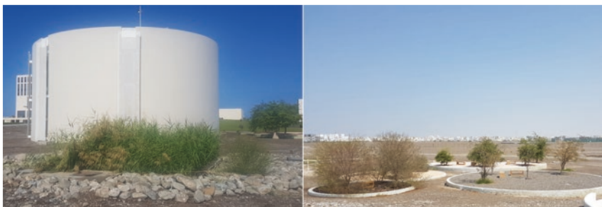
Fig. 12.1 The circle-shaped Ecohaus and the demonstration horizontal flow CW for onsite wastewater management and the reuse irrigation field at the the German University of Technology in Oman
