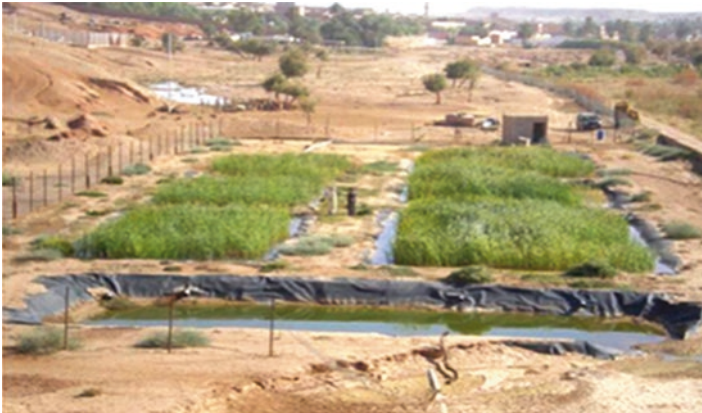
Fig. 2.2 Constructed wetlands of Brézina Oasis (October-2013) [17]
