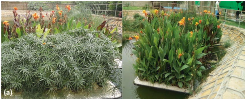
Fig. 13.3 A floating CW for retrofitting a pond system treating sewage in Karachi, Pakistan. (Photo courtesy A. Mustafa)
