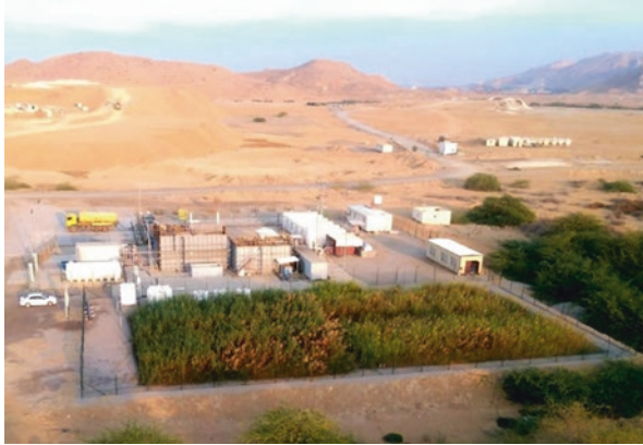
Fig. 12.2 Aerial view of the experimental VFCW system in Quriyat, Oman
