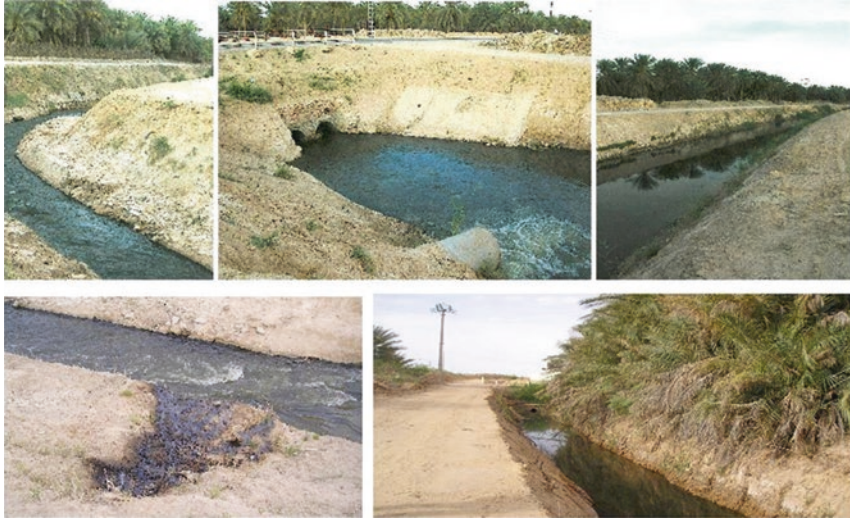
Fig. 20.7 Photos of the area's date palm plantation drainage channel increasingly used as sewage and general pollution sink, Tamacine, Algeria (field visit 2006)
