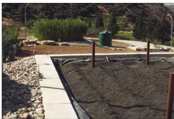
Fig. 11.6 The two-stage treatment wetland, first stage (single-pass) and second stage (planted bed) at the site
