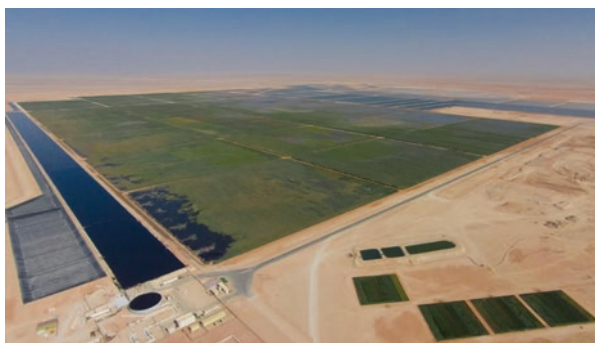
Fig. 12.5 Aerial view of the Constructed Wetland facility for oily produced water treatment in Oman. (Courtesy: Bauer Resources GmbH)
