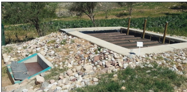
Fig. 11.3 The VFF with the flow splitting-box at Fuhais, Jordan
