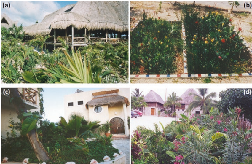
Fig. 20.3 Yucatan coastal Wastewater Garden systems: (a) Xpu-Ha Ecopark beach restaurant (b) ecological field station, Akumal (c) house Akumal (d) WWG in front of Italian restaurant/resort, Tulum
