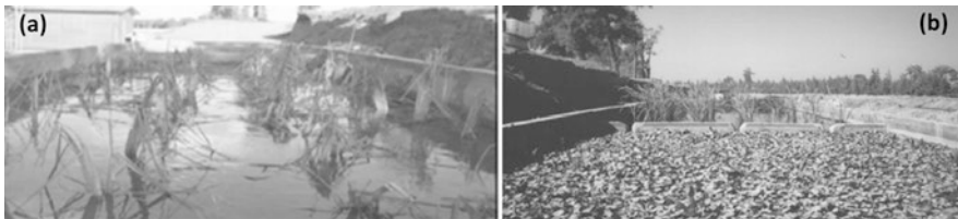
Fig. 5.12 Combined system of FWS and FAP CWs for drainage water treatment; (a) FWS and (b) FAP units [51]
