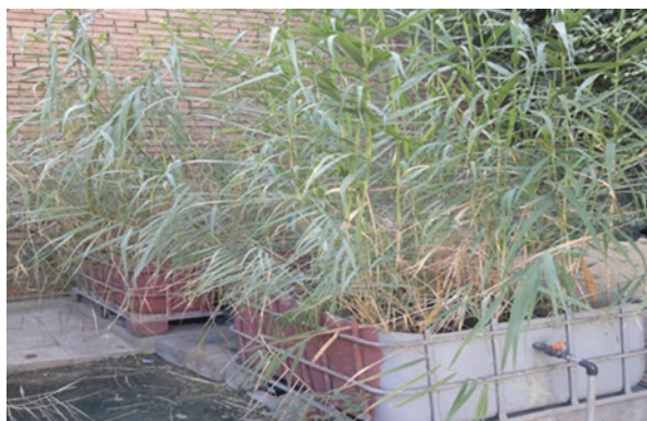
Fig. 5.16 A pilot plant comprising of a sedimentation tank followed by a hybrid CW (HSSF and VFCW) for greywater treatment [58]
