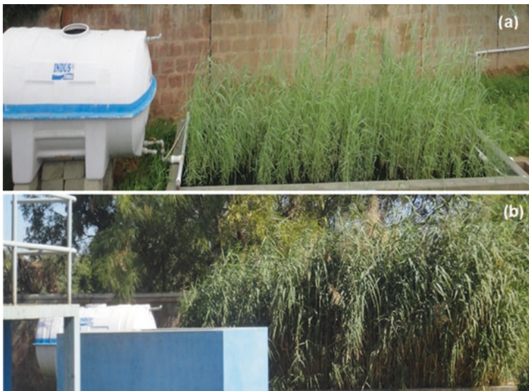
Fig. 13.1 A pilot-scale horizontal surface flow constructed wetland in Karachi for effluent reuse (a) during plant establishment period (b) after establishment period. (Photo courtesy A. Mustafa)
