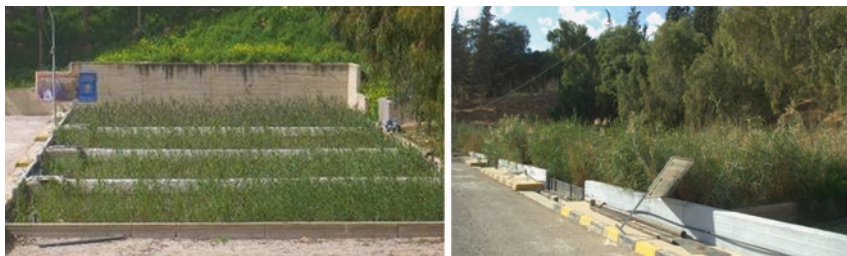
Fig. 15.7 STW beds in Al-Salt wastewater treatment plant in Jordan [43, 44]
