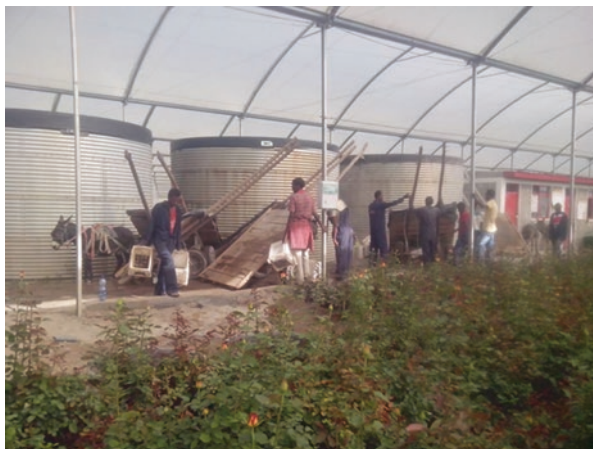
Fig. 7.2 Building of the first wetland, donkeys at the vocom. (Photo: ECOFYT ©)
