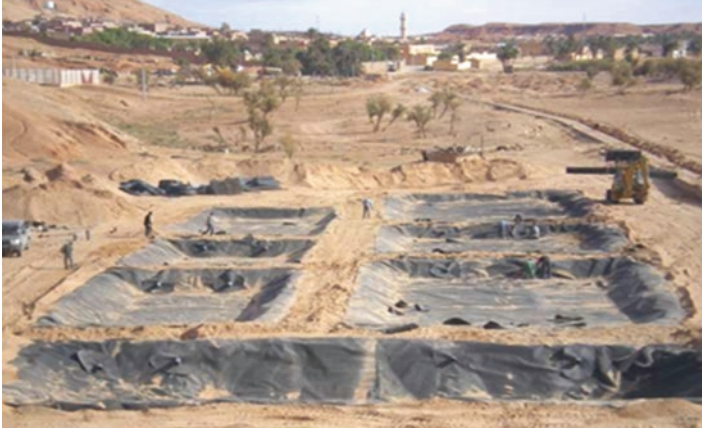
Fig. 2.1 View of the Constructed wetlands of Brézina Oasis under construction [42]
