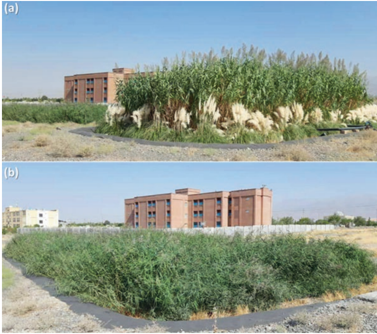
Fig. 14.3 Pictures of (a) the VFCW bed and (b) the HFCW bed of the hybrid CW system at the Neyshabor University
