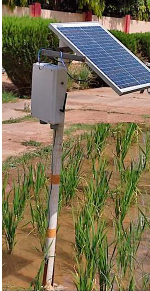
Fig. 2. Installation site of LoRa based sensor node.
