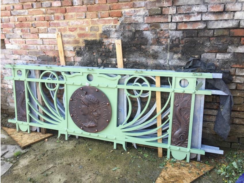
Fig. 10. Application of the overall system of corrosion protection to the Čech Bridge railing segment
