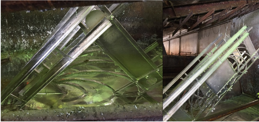
Fig. 9. Demonstration of hot dip galvanizing application.
