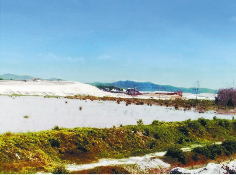
Fig. 7.2 Tin tailing dump in Thailand – tailings are stored in impounded dams (after Yap 2007) and in the background is a coarse sandy tailing stockpile where very little vegetation will grow due to nutrient limitations despite the high prevailing tropical rainfall conditions
