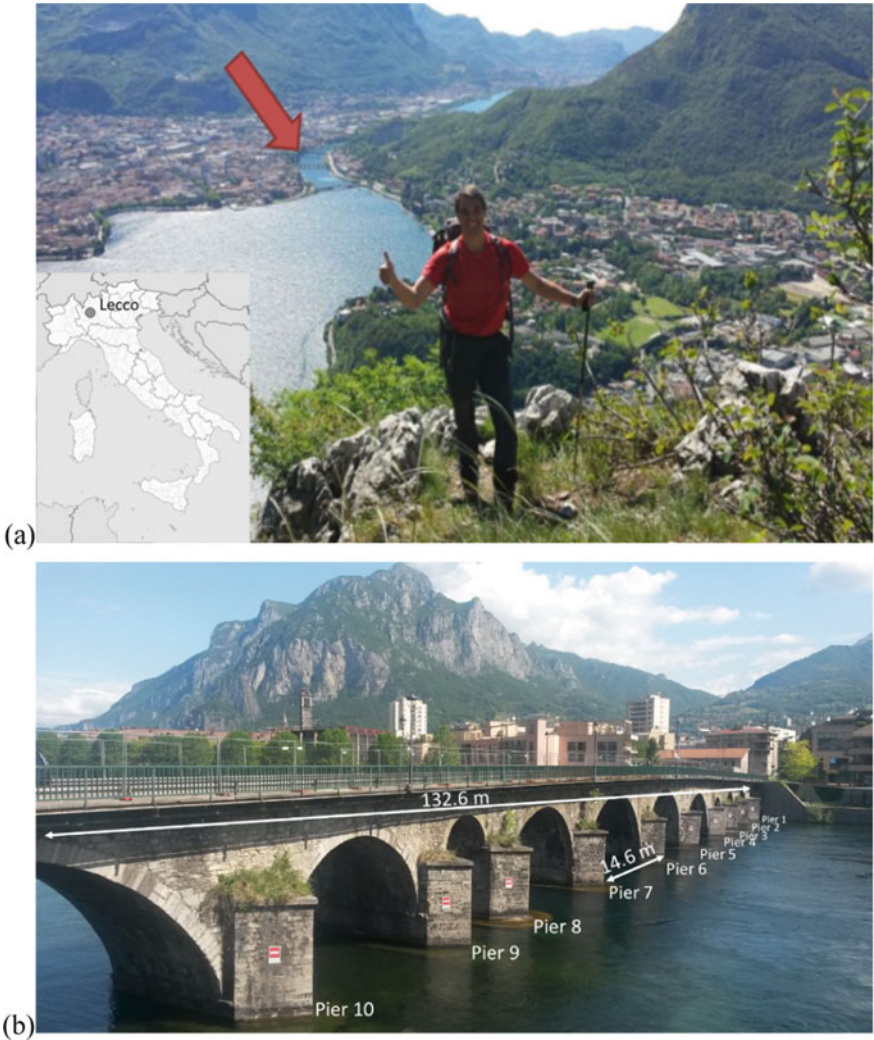
Fig. 4 a position of the town of Lecco in Italy and panoramic view of the lake of Lecco and of the location of the Azzone Visconti bridge; b view of the Azzone Visconti bridge in 2014, at the beginning of the investigation campaign
