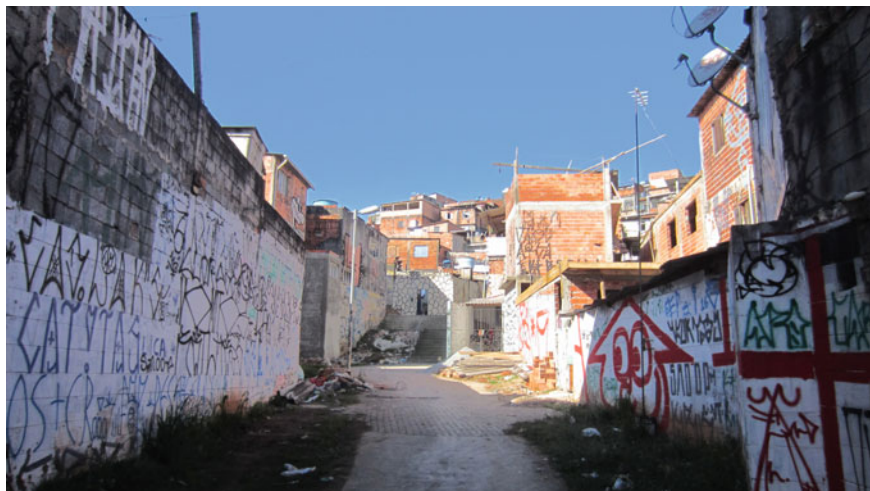
Fig. 13.2 Section 1 of the Green Path. Pedestrian walkway over the stream bed, lined by the back walls of houses. Photo Solange Carvalho
