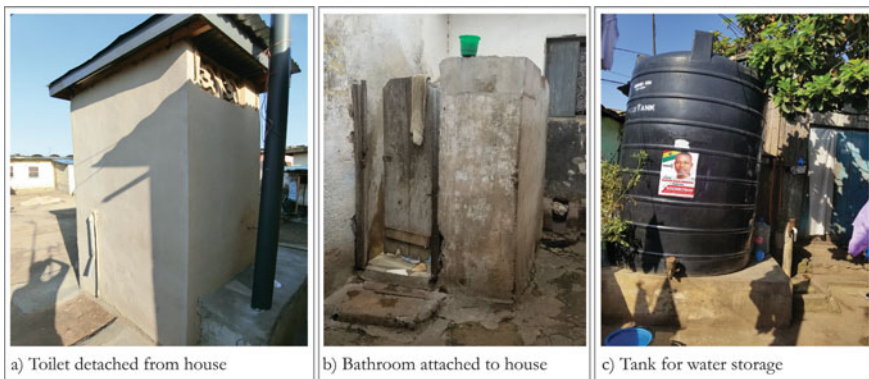
Fig. 37.4 Sewage and drainage conditions. Photos Okyere, Diko, Ebashi, Kita
