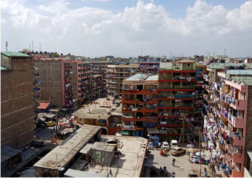
Fig. 42.7 Section of Pipeline Estate. Photo Edwin Oyaro Ondieki
