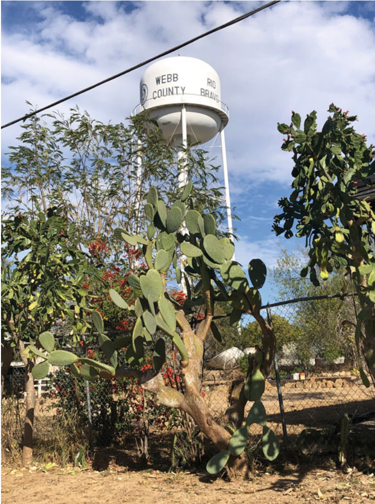
Fig. 20.1 Rio Bravo water tank. Photo Emilio Longoria
