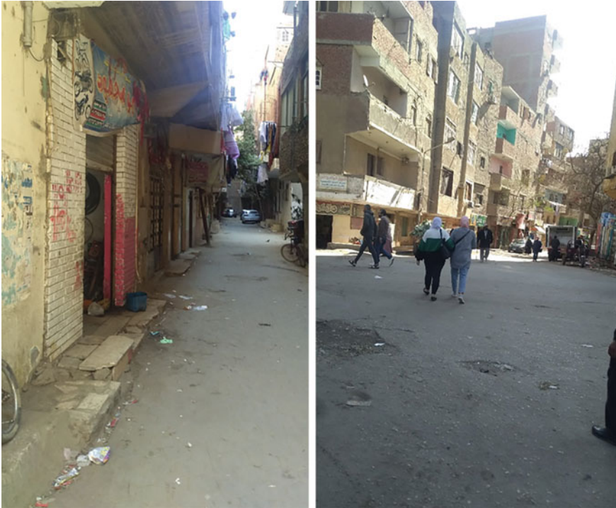
Fig. 35.5. Poor maintenance of upgrading projects in Giza Governorate
