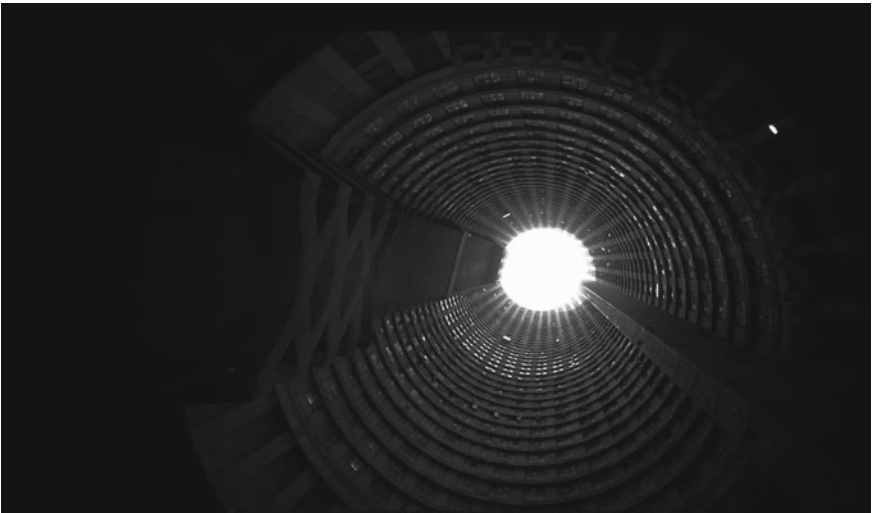
Fig. 41.2 Utopian city-within-a-city, Ponte City. Photo Gregory Marinic
